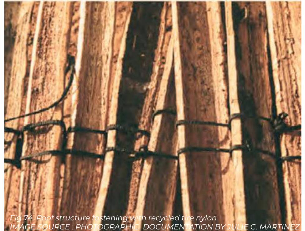
Fig 74. Roof structure fastening with recycled tire nylon
