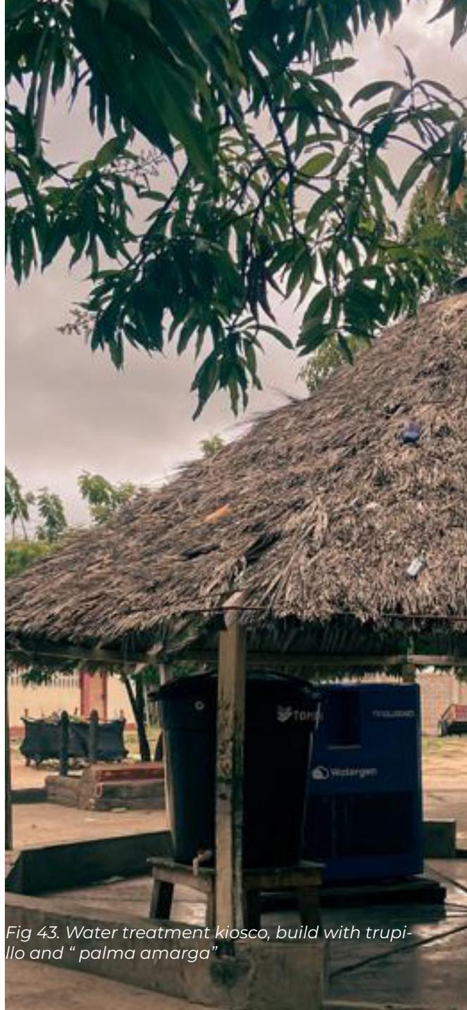
Fig 43. Water treatment kiosk, build with trupi-
