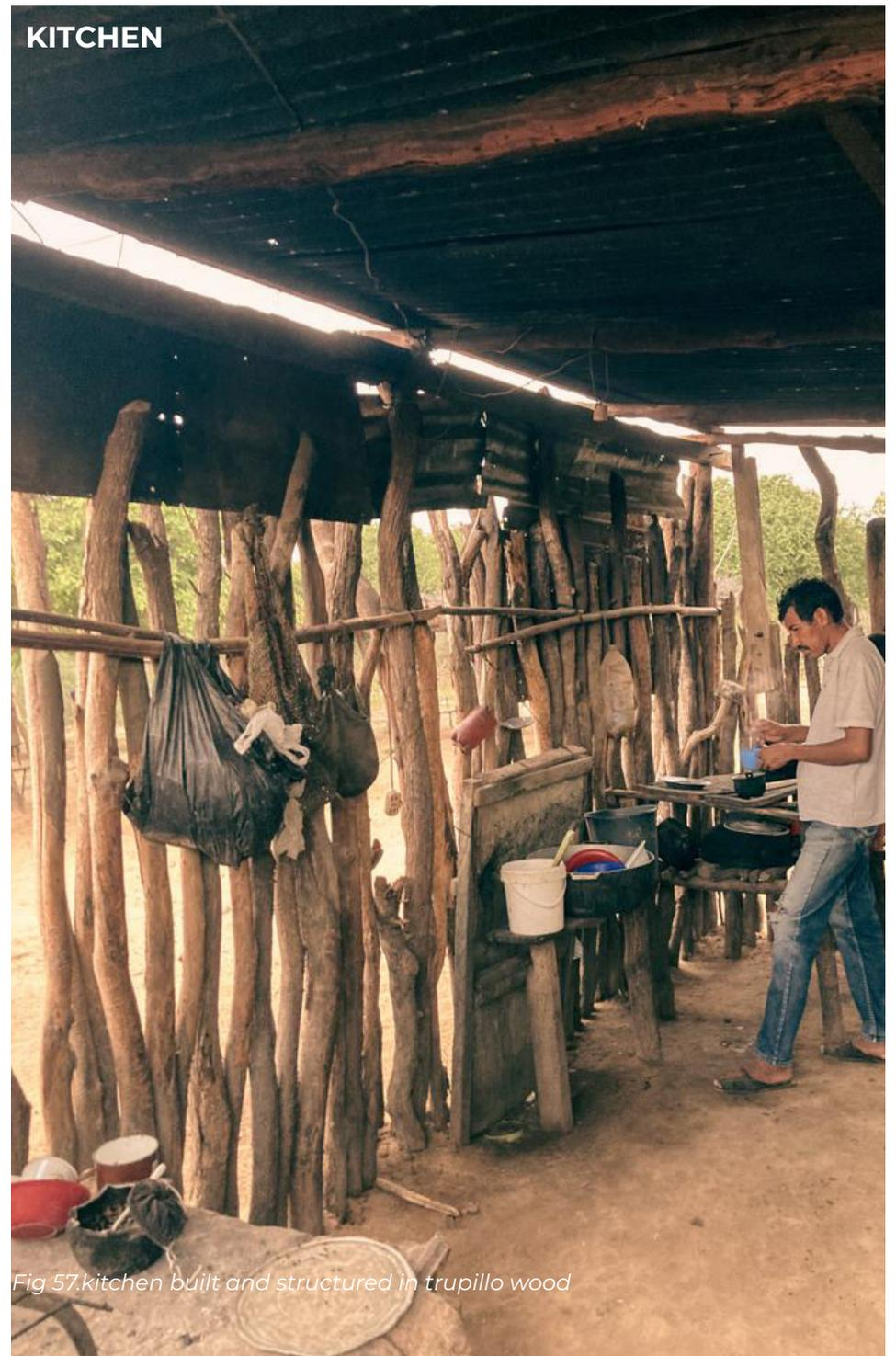
Fig 57.kitchen built and structured in trupillo wood
