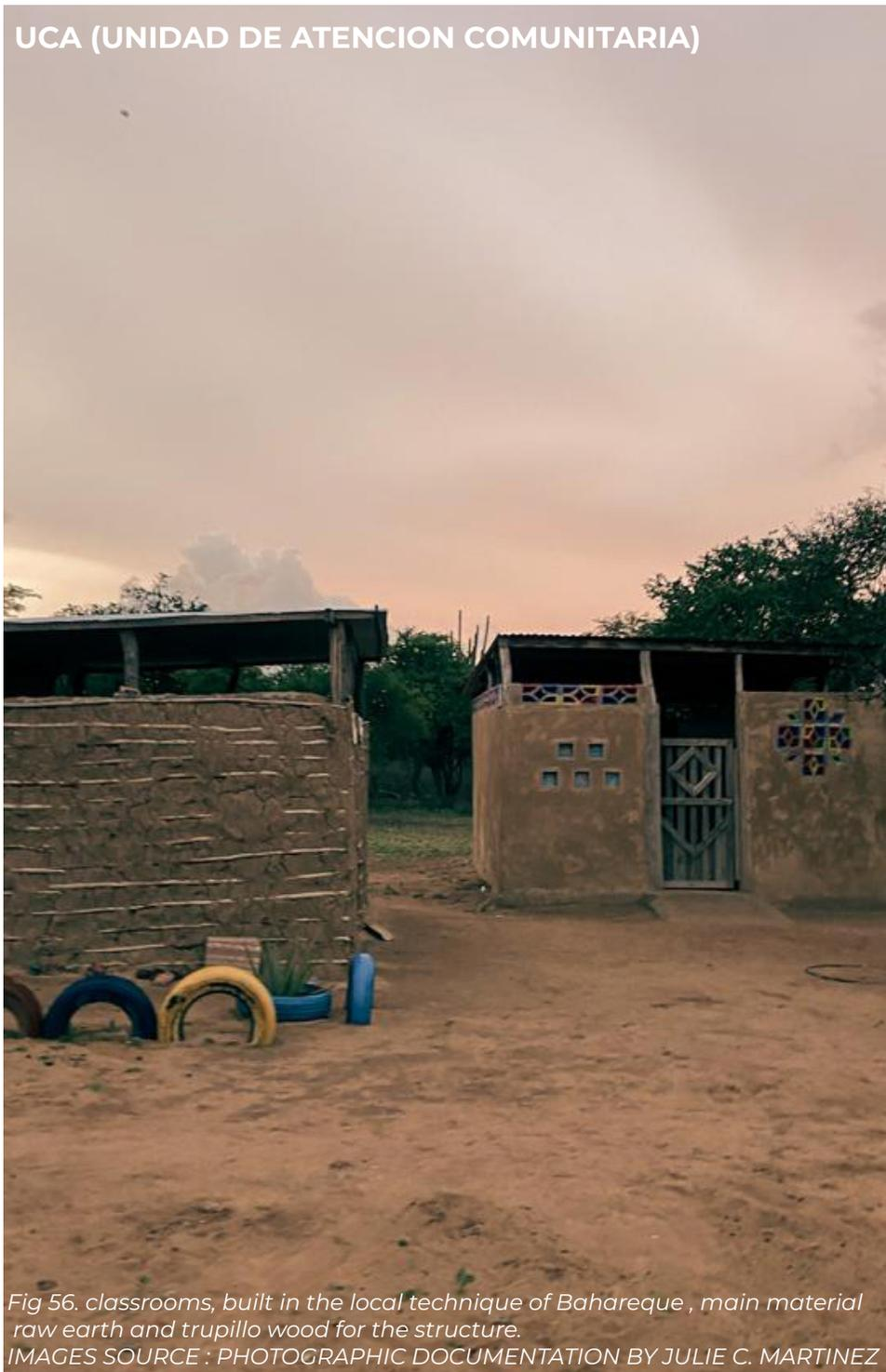
Fig 56. classrooms, built in the local technique of Bahareque , main material raw earth and trupillo wood for the structure.
