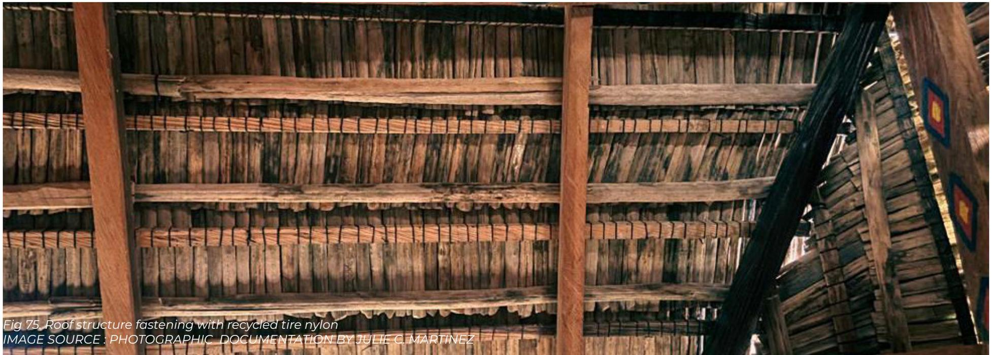
Fig 75. Roof structure fastening with recycled tire nylon
