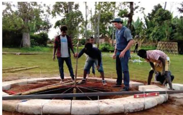
Figure 67: Circular fondation made of stone blocks
