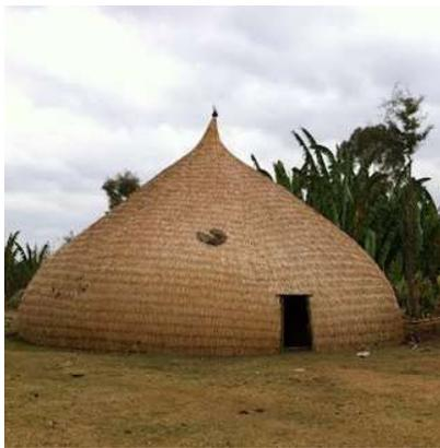
This is a traditional cut and braided bamboo circular house made by the Sidama people of Ethiopia. The dome, with its pointed top, is designed to repel heavy rain while in a circular dome that space would have a flat area, prone to leaks.
