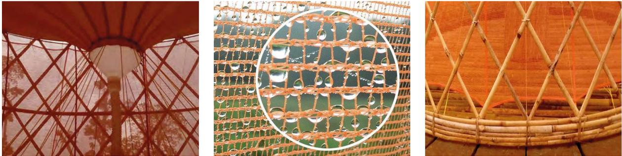
Figure 62: Water is collected from rain, fog and dew. the polyester net membrane captures water, filters and channels it into a 3000 litres water collection PVC tanker.
