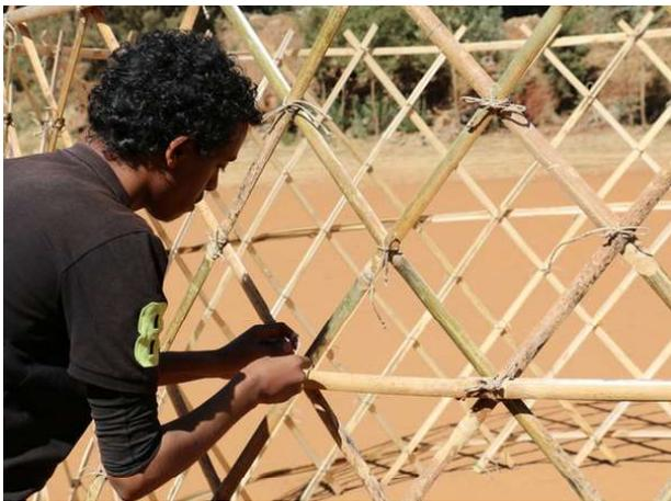
Figure 65: Work in Progress - WW 3.2 - First Test Assembly with hemp ropes
