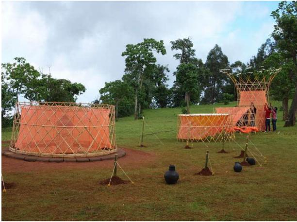
Figure 64: Five modules are layered from top to bottom and connected to each other using natural fibre ropes
