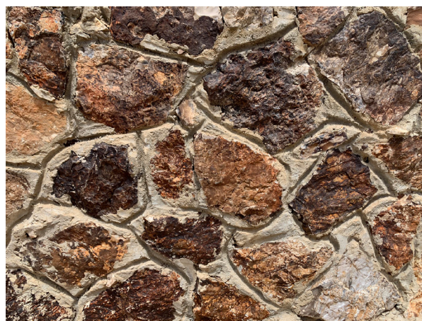
Fig 69. Partition built of Arad stone, carved into irregular, pointed stone fragments, 2022. Source: the author.
