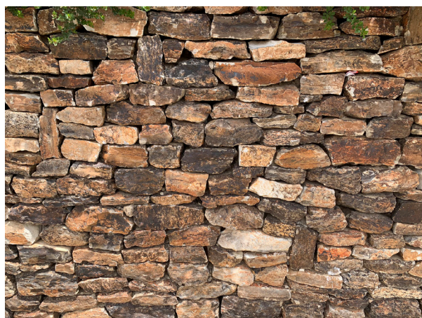
Fig 68. Wall of interlocking Arad stones, hewn similarly to standard building bricks, 2022. Source: the author.
