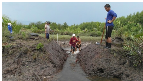
Figure 43 Adjusting hydrology – by digging channels to improve water flow (Source- https://mangroveactionproject.org/mangrove-restoration/ )
