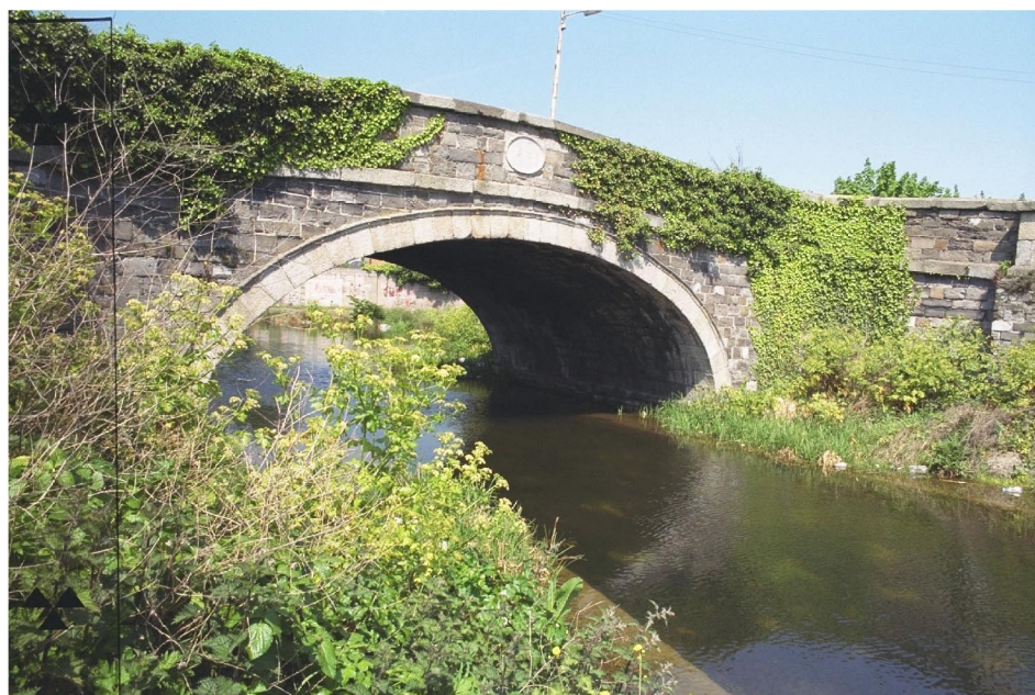
Fig. 2 A typical masonry arch bridge, Griffith Bridge, Dublin, Ireland
