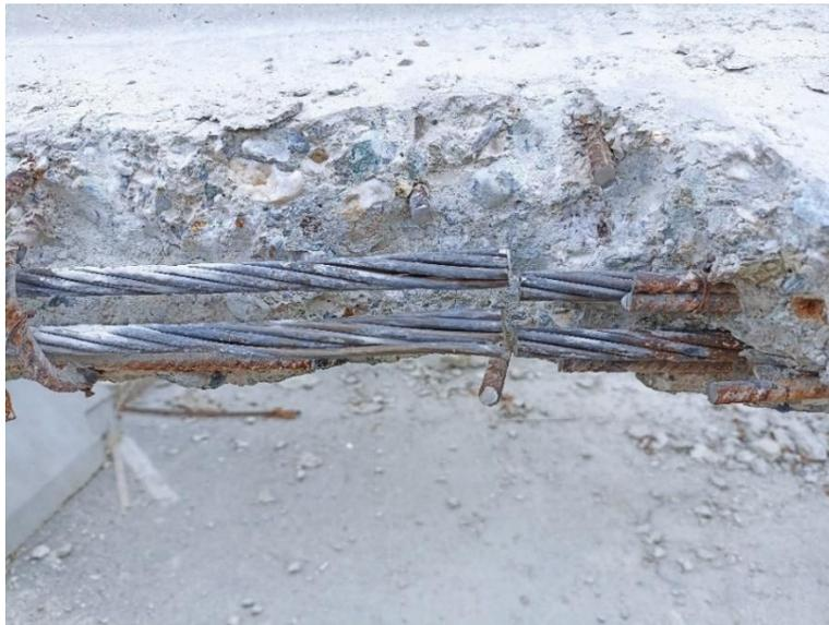
*Figure 32. Completely cut strands.*
