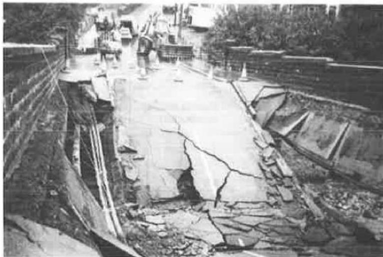
*Figure 6. Ynys-y-Gwas bridge after collapse, West Glamorgan, UK (Woodward, 1989).*
