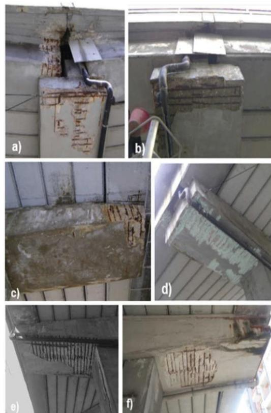
*Figure 8. Degradation and corrosion at support zones in the Corso Grosseto viaduct at different years of inspection. a) 2011, b) 2012, c) 2013, d) 2014 maintenance interventions, e) 2015 and f) 2016. (Savino et al., 2021)*
