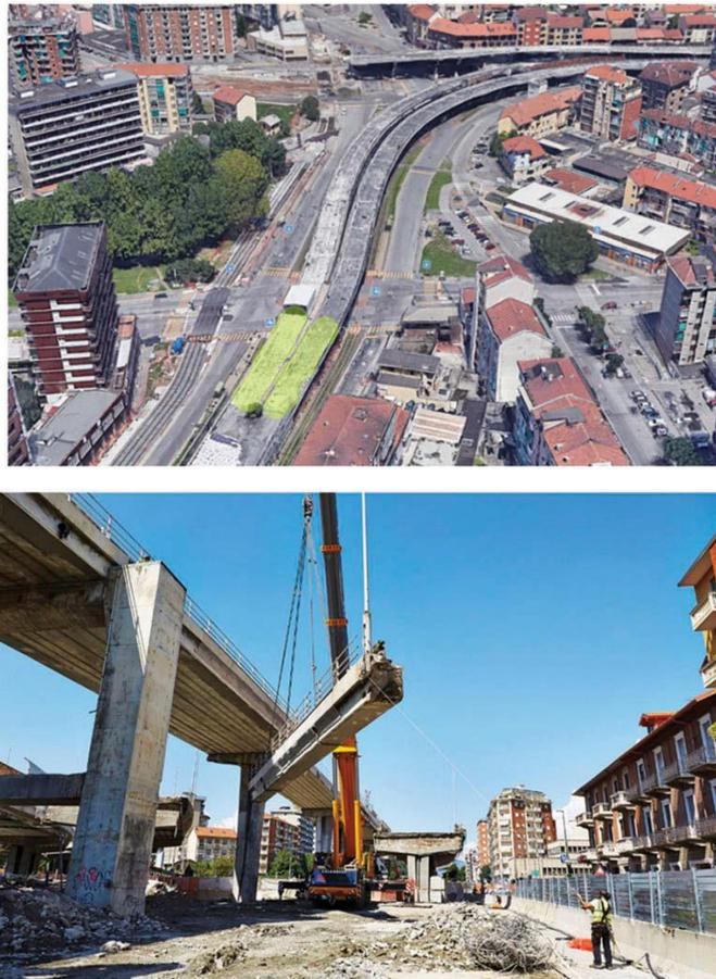
Figure 1. (a) Corso Grosseto viaduct (Turin). (b) Bridge deconstruction process (Anghileri, Biondini, et al., 2021).
