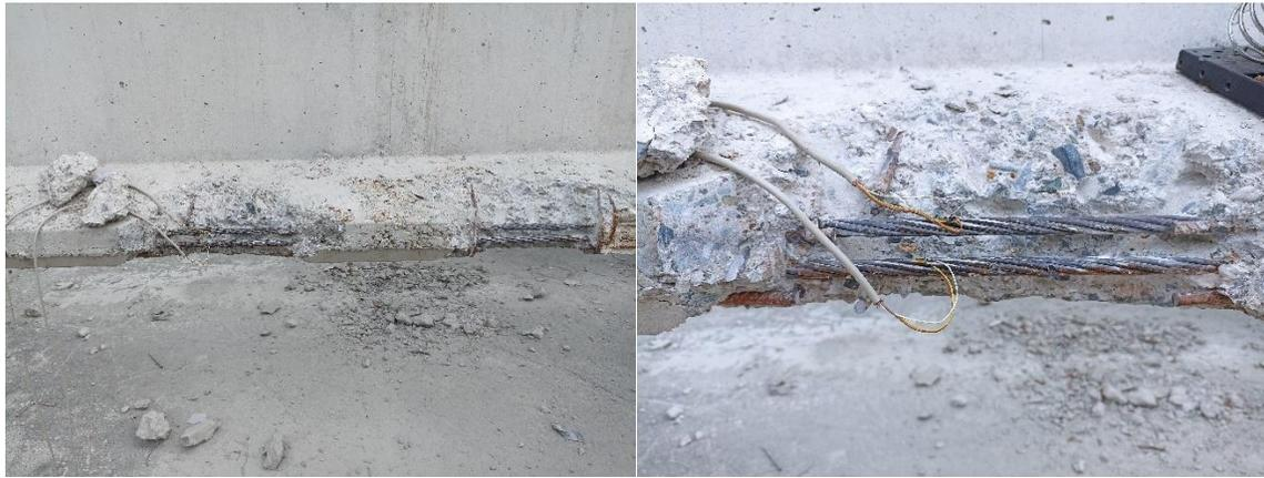
*Figure 31. Configuration before strand cutting.*
