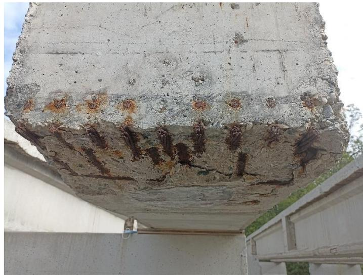
*Figure 4. Prestressed corroded tendons at the end of a PC beam.*
