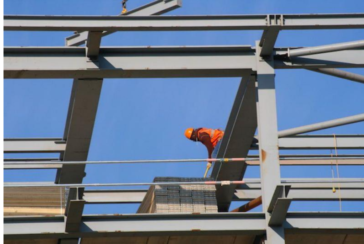
Figure 120. Assembly of steel structure beams representation
