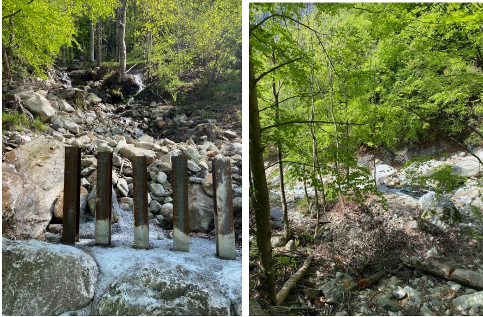
Figure 6. Defense for crosswalk and Landslide of River embankment
