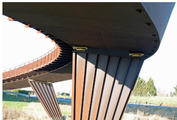
Figure 22. Shanks Millennium Bridge Peterborough, England.
