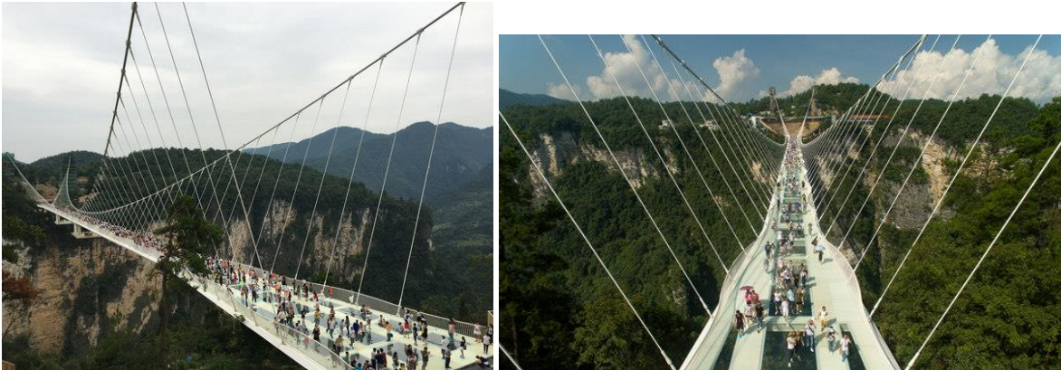
Figure 16. ZHANGJIAJIE GRAND CANYON GLASS PEDESTRIAN BRIDGE
