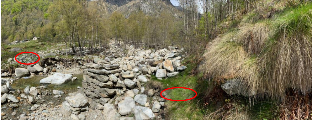
Figure 24. Position Piles and Foundations for new pedestrian bridge
