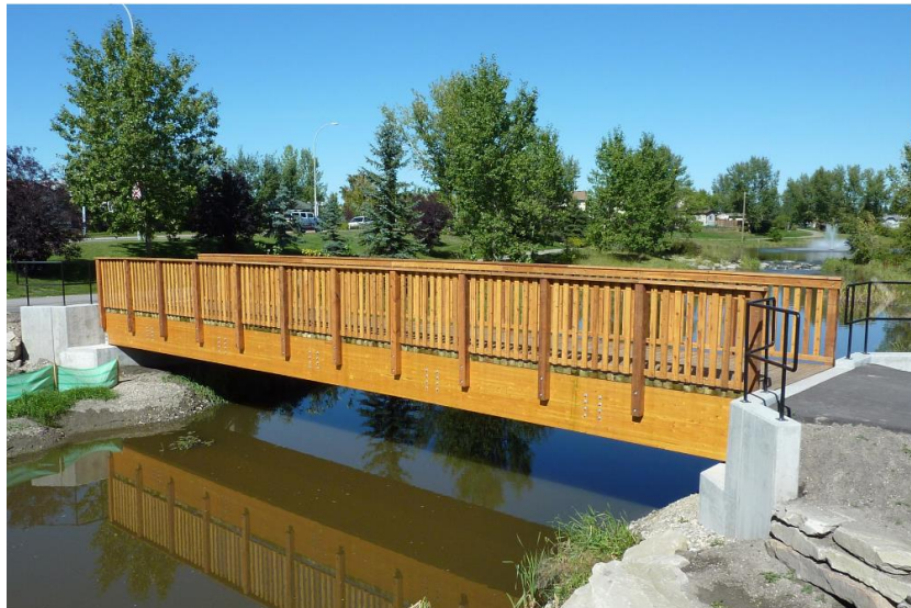
Figure 27. Glulam Beam Pedestrian Bridges (Taken from Custom Park & Leisure Ltd.)
