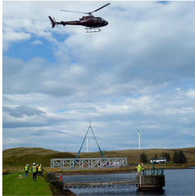
Figure 112. Representation of transport of steel materials by helicopter (CTS bridges limited. (s.f.). “FRP bridges installed by helicopter – Scotland”)
