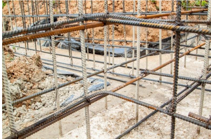
Figure 118. Assembly of reinforcement steel for foundation representation
