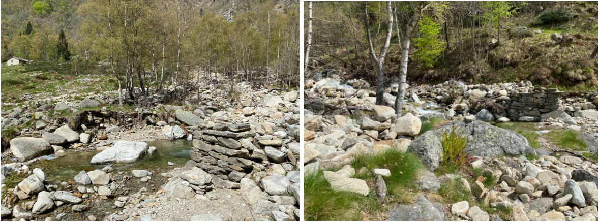
Figure 2. Actual aspect of pedestrian bridge in Valle Mologna
