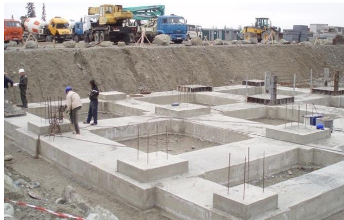
Figure 119. Foundation cast in place concrete representation
