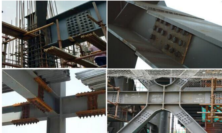
Figure 121. Assembly of steel structure connections representation
