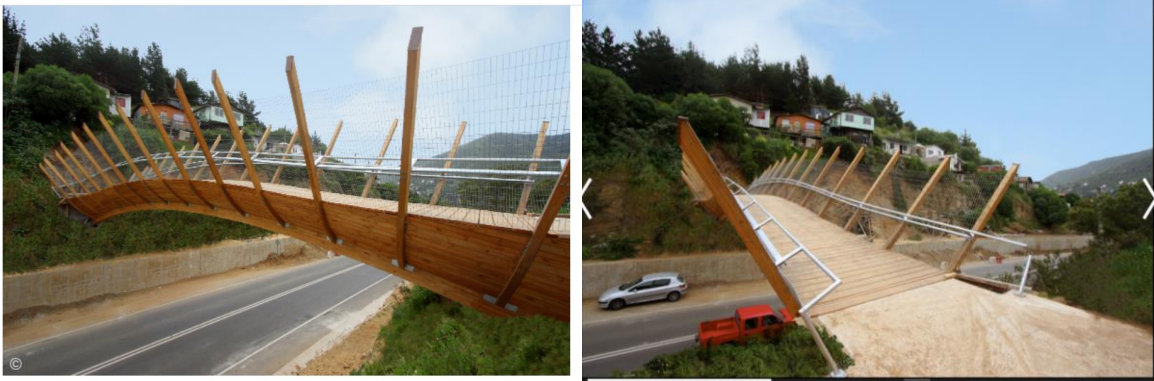
Figure 12. Zapallar Pedestrian Bridge
