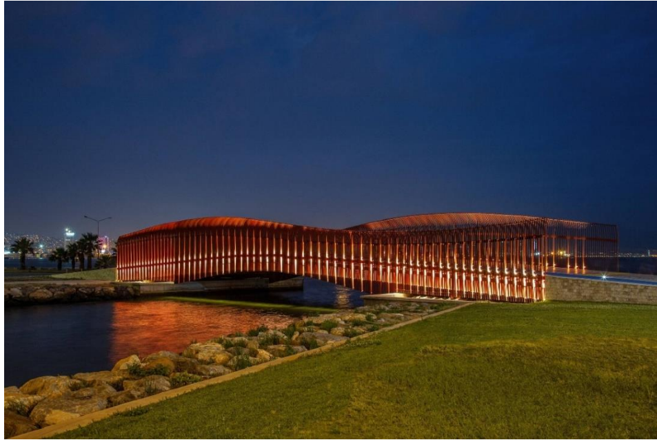
Figure 173. Bayrakli Coast Pedestrian Bridge at night (Taken from Archdaily.com)
