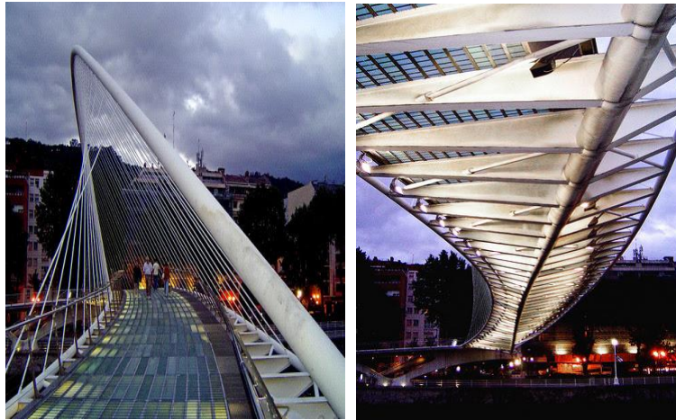
Figure 15. Campo Volantin PEDESTRIAN BRIDGE
