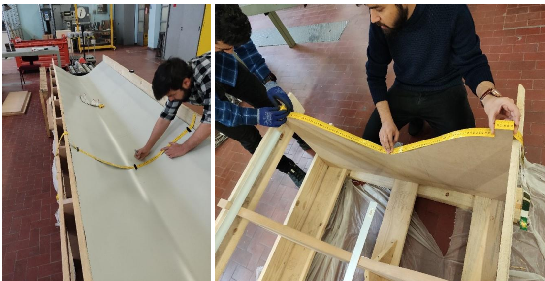
Figure 68 marking the diaphragm and placing the sheet with nails.
