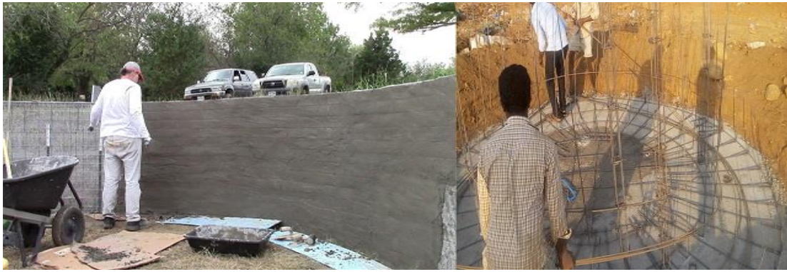
Figure 8 ferrocement walls and shell in India [9]
