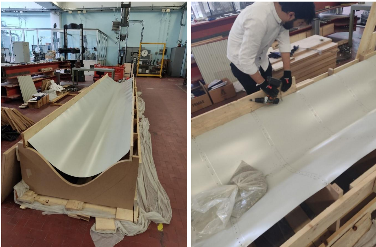
Figure 66 placing steel sheet
