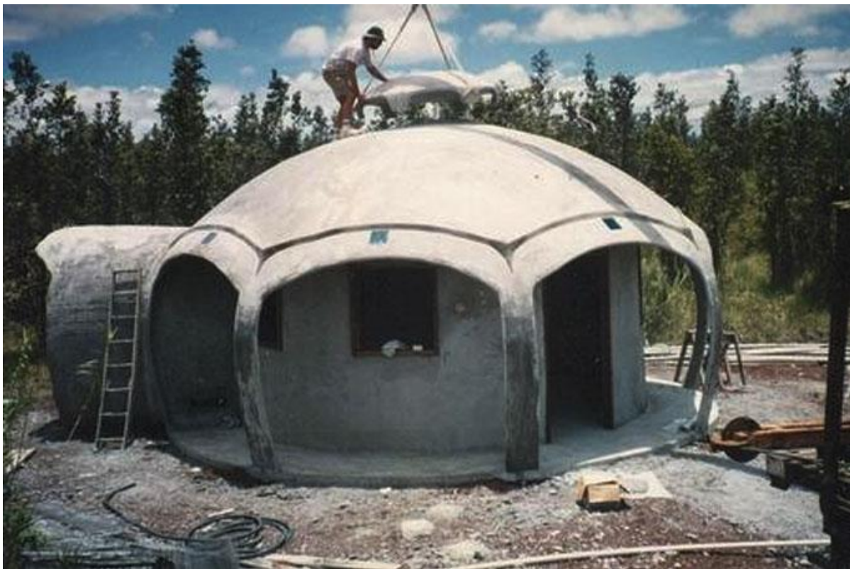
Figure 9 ferrocement dome shaped house [7]
