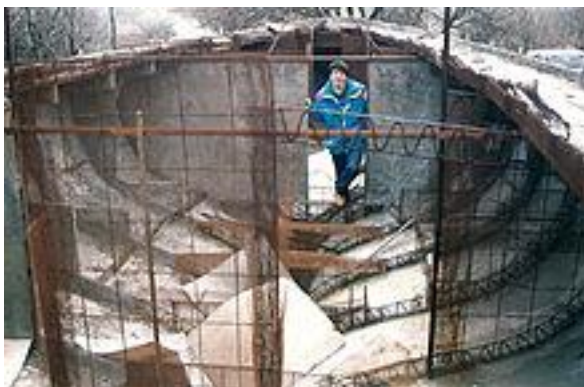
Figure 7 ferrocement wall in construction [7]
