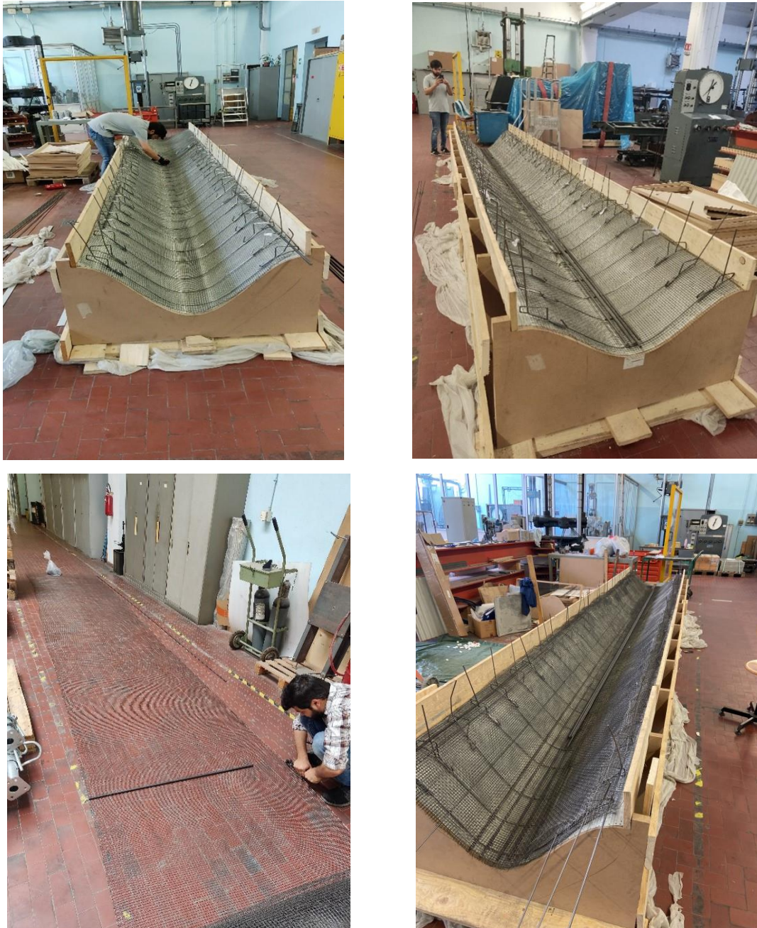
Figure 73 transversal reinforcements and longitudinal reinforcements with wire mesh layers.
