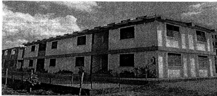
Figure 5 typical ferrocement housing units
