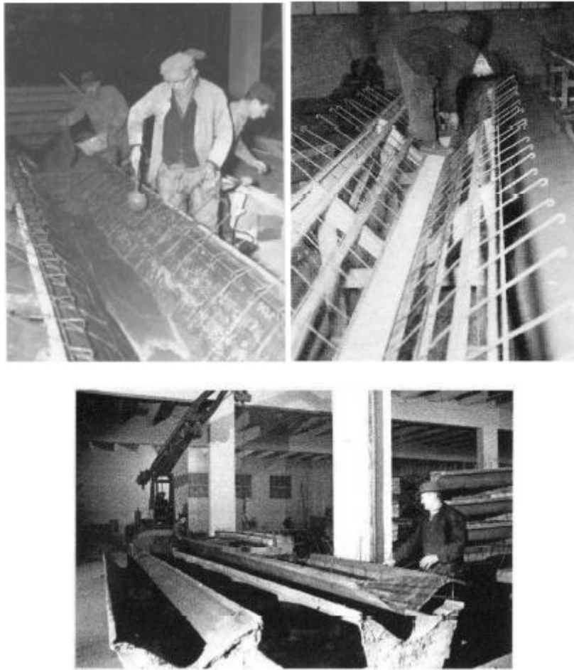
Figure 57 ferrocement realization as done by Nervi
