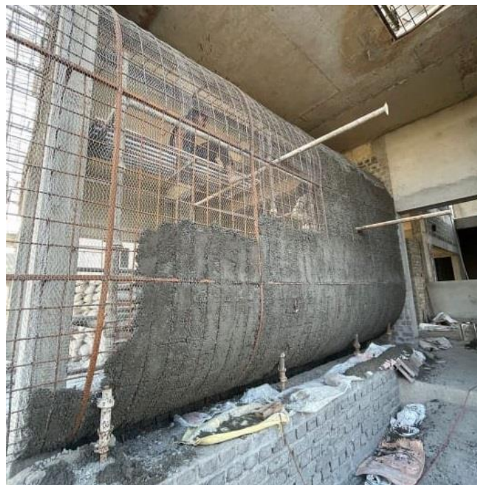
Figure 7 ferrocement wall in construction [7]
