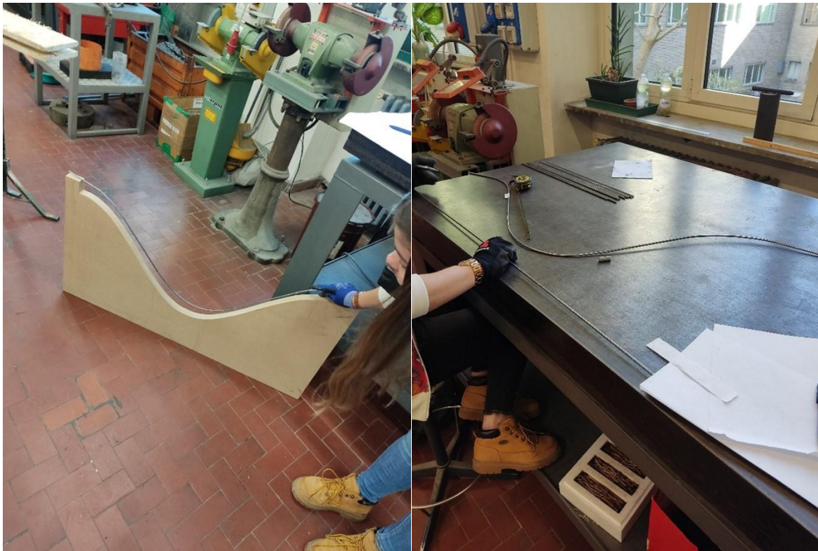
Figure 70 bending the transverse reinforcements
