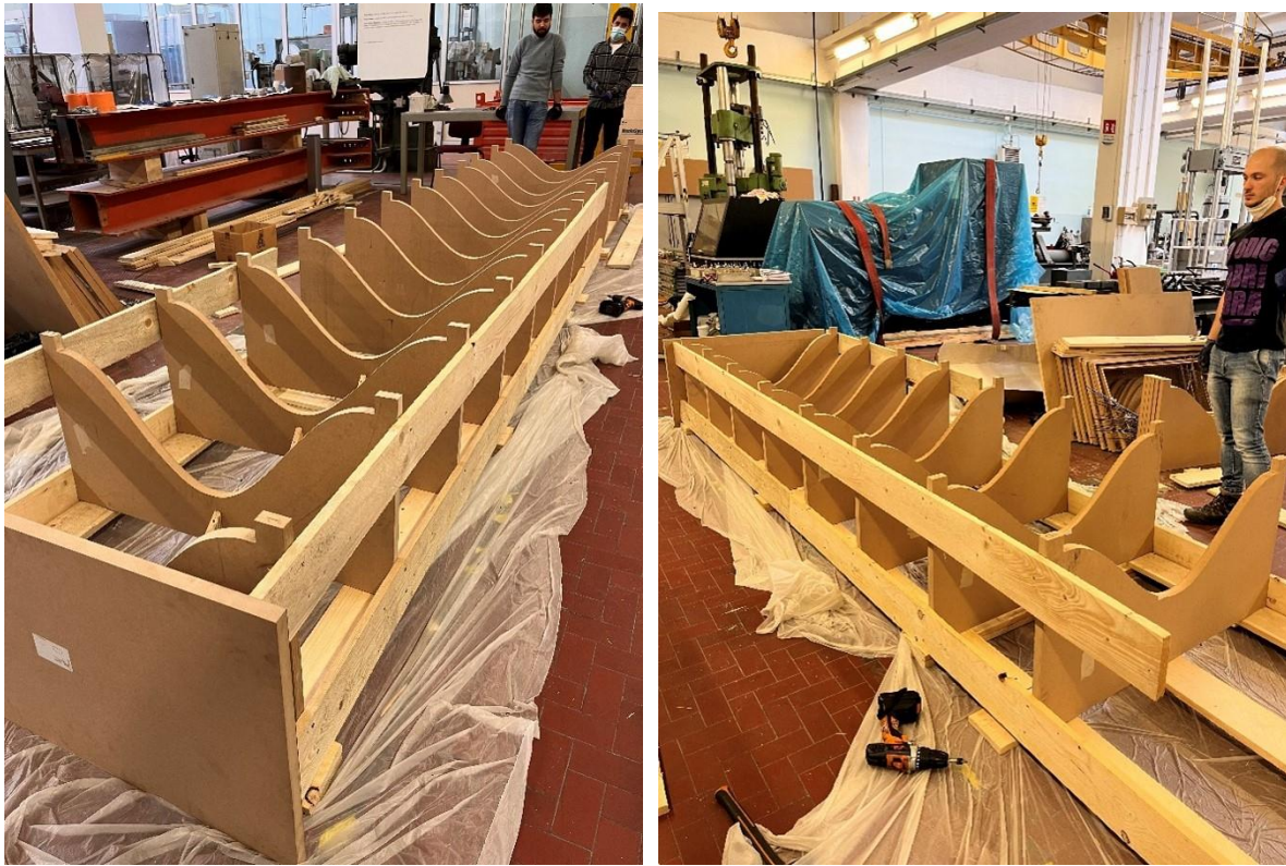
Figure 64 side rails and curved panels placed.
