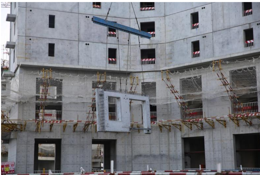
Figure 92: Prefabricated modules on site (source: https://www.gooood.cn/baiziwan-social-housing-by-mad.htm )
