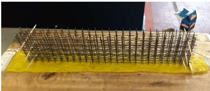
*Figure 45 Steel net with positioned wood sticks*
