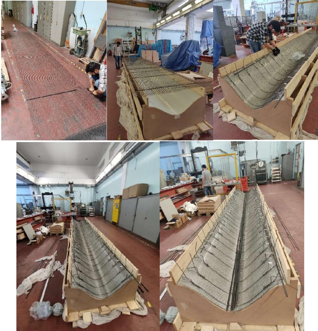
*Figure 63 Reinforcement application procedure, from high on the left side: Steel nets cutting, Steel nets straightening and positioning, transversal reinforcement positioning and fixing, transversal reinforcement positioned, longitudinal lower reinforcement application*
