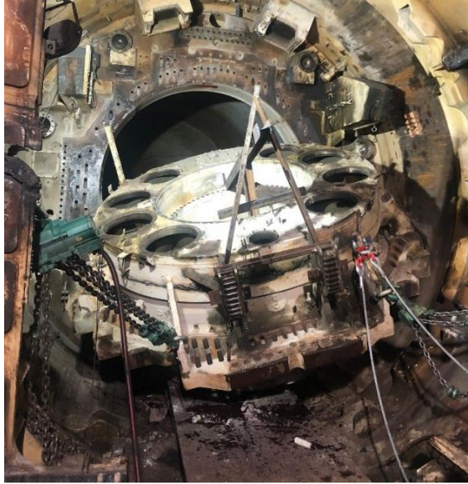
Figure 41- main drive lying on the shield floor, trolley and easel devices
