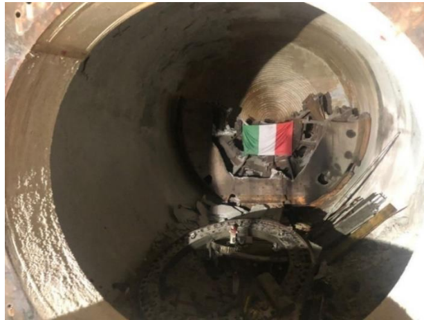
Figure 33 - Cutterhead divided into three portions. The photo was taken after the main drive disassembly
