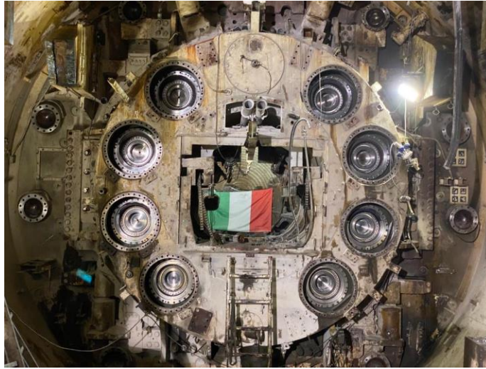
Figure 37 - disassembly of the shield area: removal of main thrust cylinders, gripper cylinders, torque cylinders and electromotors with gearboxes
