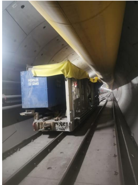
Figure 34 - example of gantry transportation (gantry 24)
