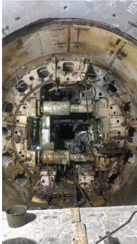
Figure 36 - disassembly of the shield area: removal of thrust cylinders
