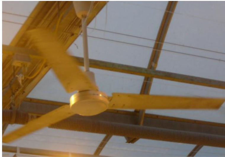
Figure 6.9: Paddle fan to increase vertical air movement and therefore evapotranspiration. This is important for the prevention of tipburn.
