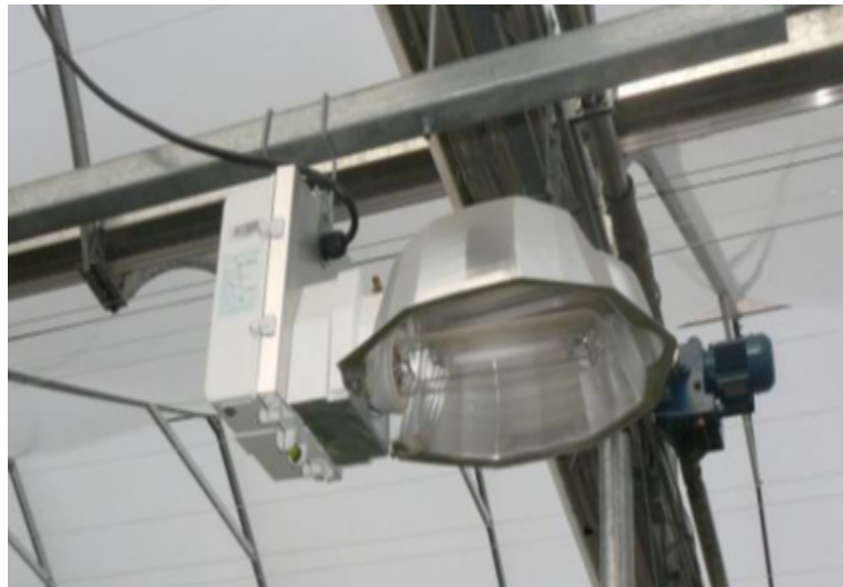
Figure 6.7: High Intensity Discharge (HID) luminaire in a greenhouse.
