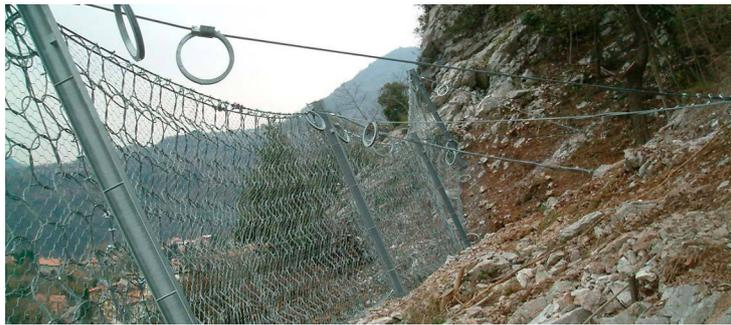
Figure 1.10: Example of a rockfall barrier (picture taken from [4])
