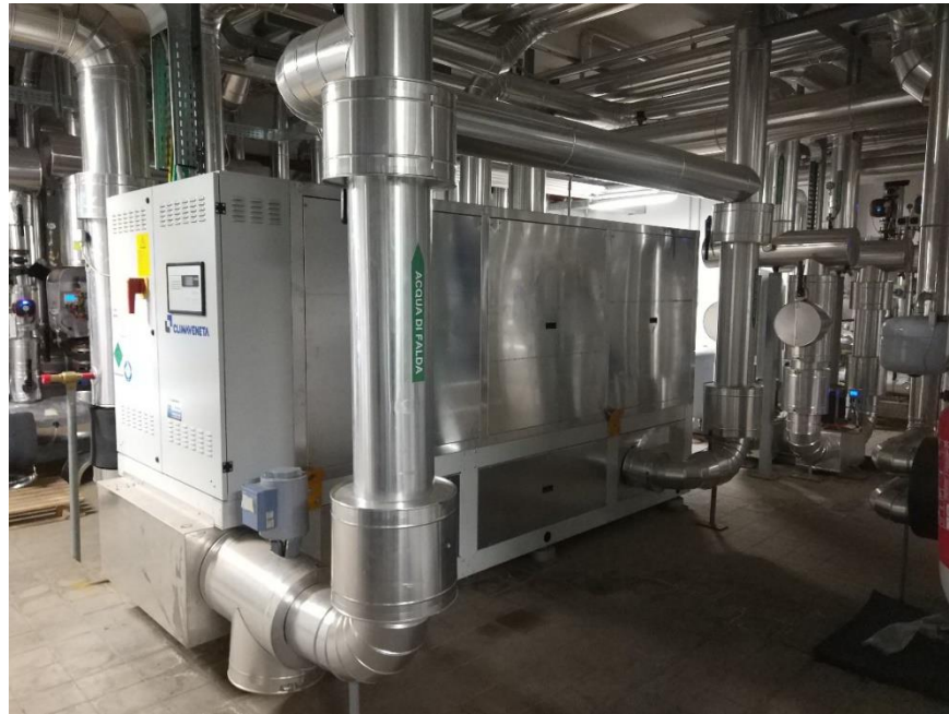
Figure 3: Geothermal Polyvalent Group Installed in Energy Center.
