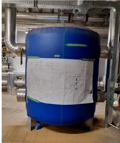
Figure 5: Thermal Energy Storage
