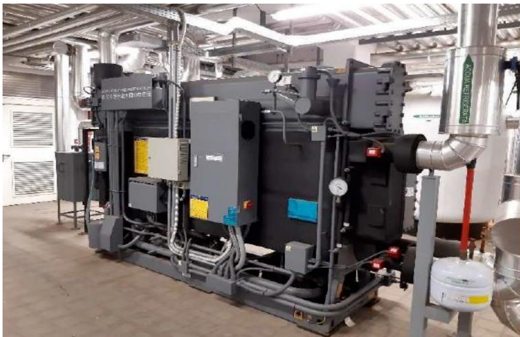
Figure 4: Absorption Chiller
