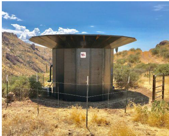
Figure 41 Arizona National Scenic Trail (AZT) Remote Rainwater Collector
