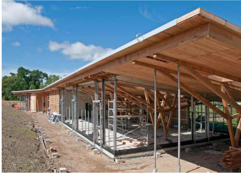
Fig. 37 Construction site Source: Architecture & Design Scotland
