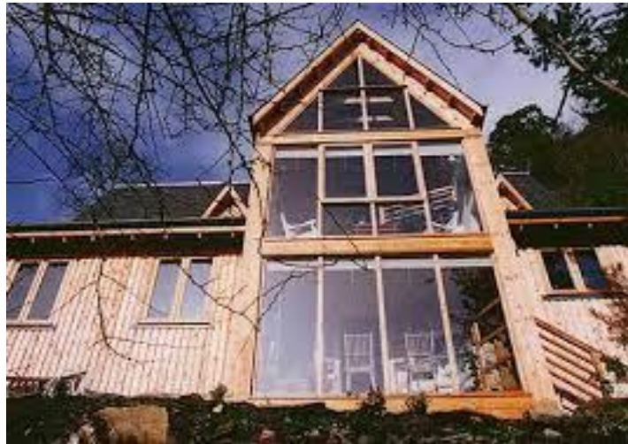
Fig. 13 Glass façade Source: GAIA Architects
