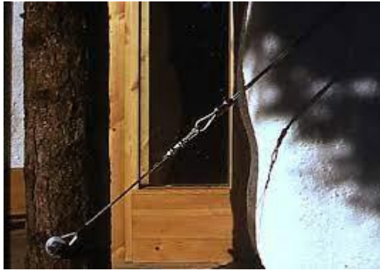
Fig. 9 Shipping fixings Source: GAIA Architects
