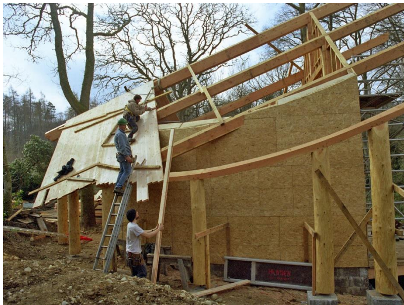
Fig. 29 Construction process Source: Robin Baker
