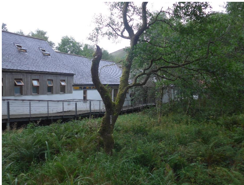
Fig. 23 Note the open skylights
