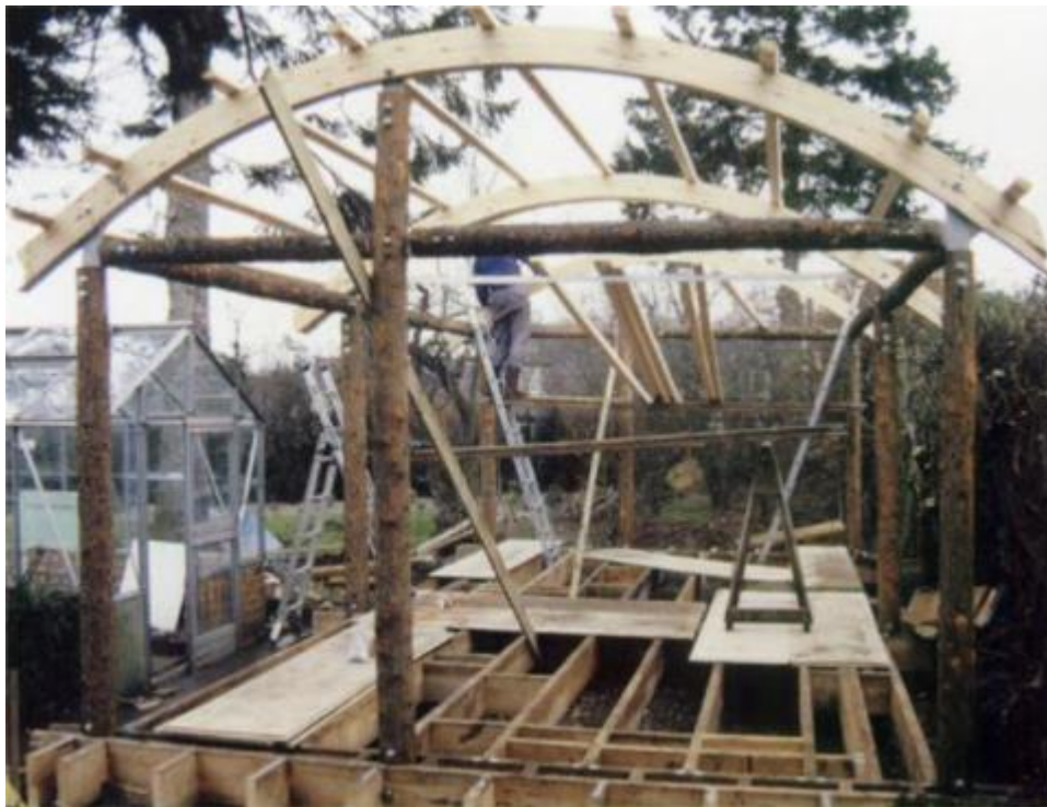
Fig. 6 Construction of the round pole structure Source: Locate Architects
