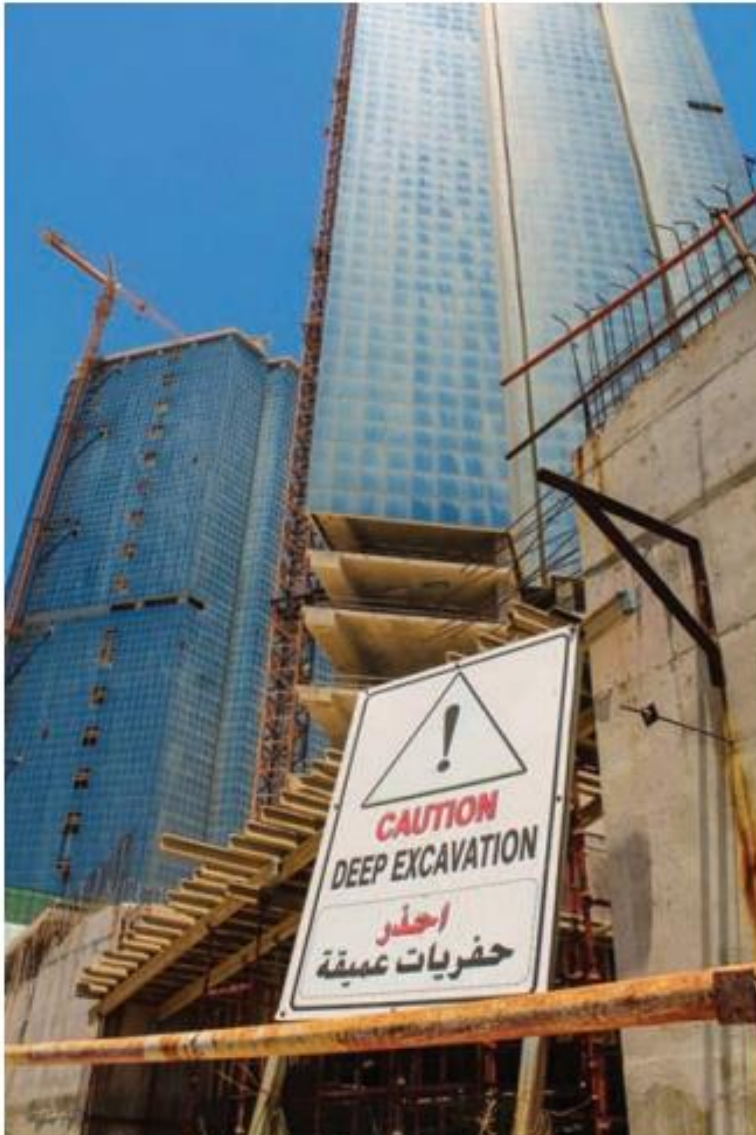
Figure 22: The Abandoned project site
