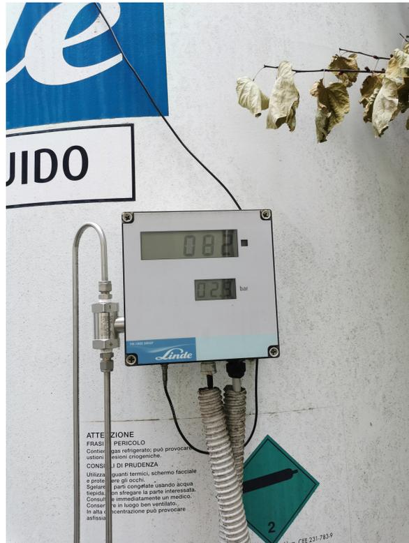
Figure 2.20: Level and pressure indicator of the tank
