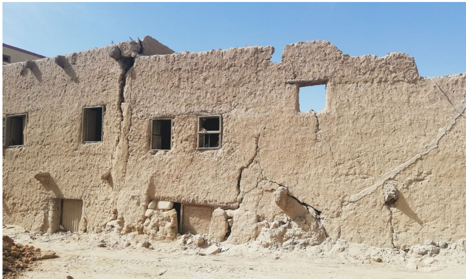
Fig. 33: Sinking house due to structure deficiency. Taken by Youssef Mekael, 2021
