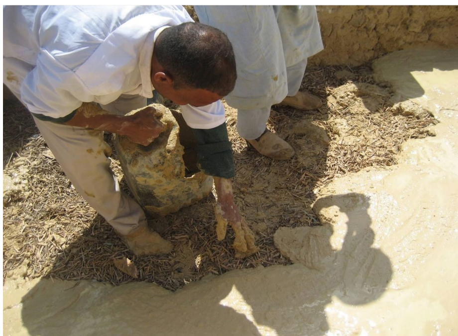
Fig. 19: Finishing layer of the roof. Taken by Emad Farid
