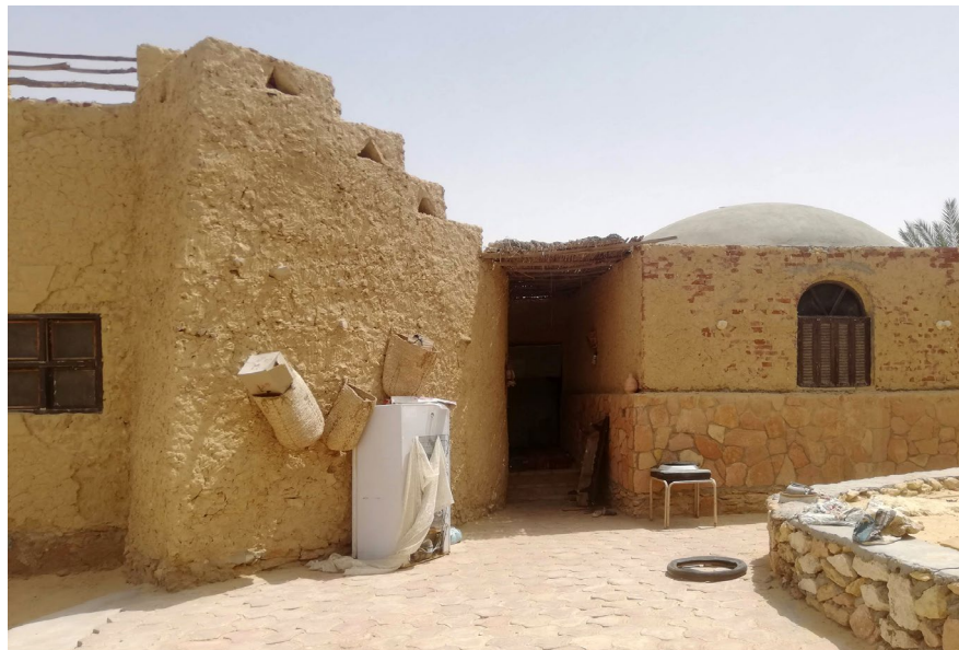
Fig. 65: A new constructed house, mixing between red bricks and Kershif. Taken by Youssef Mekael, 2021
