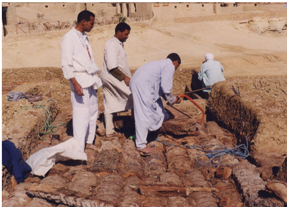
Fig. 18: Construction of the decking. Taken by Emad Farid
