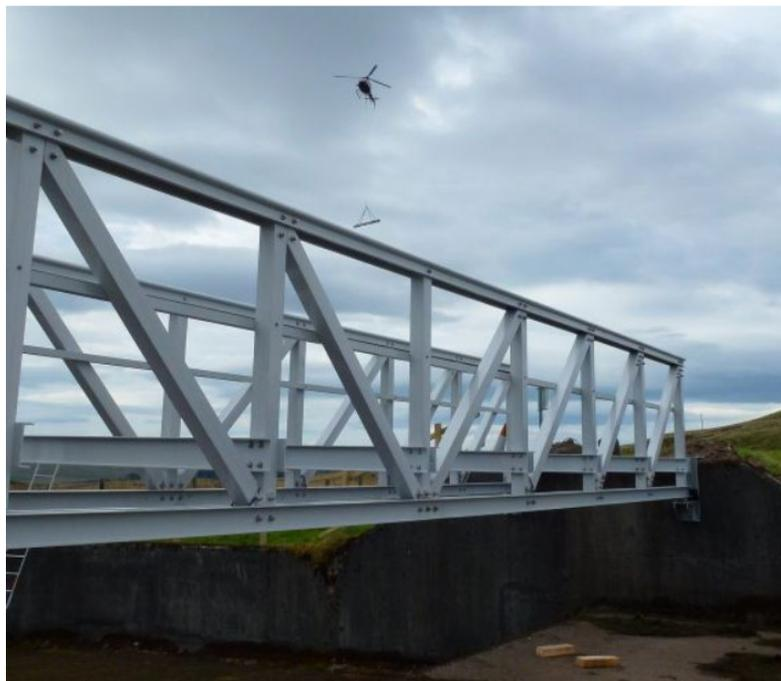
Figure 84: FRP bridge, Eastburn reservoir, Stirling - 13.5m x 1.2m; Taken from: (CTS bridges limited, s.f.)
