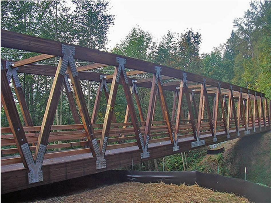
Figure 10: Bridge constructed/Taken from (Western wood structures, 2021) - Bridge made of Glulam
