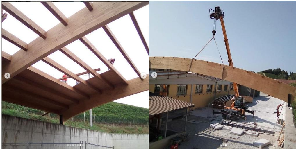
Figure 79: Cantina Beni di Batasiolo a La Morra (Cn), completed in 13 days more than 900 m2 of structure in Glulam.
