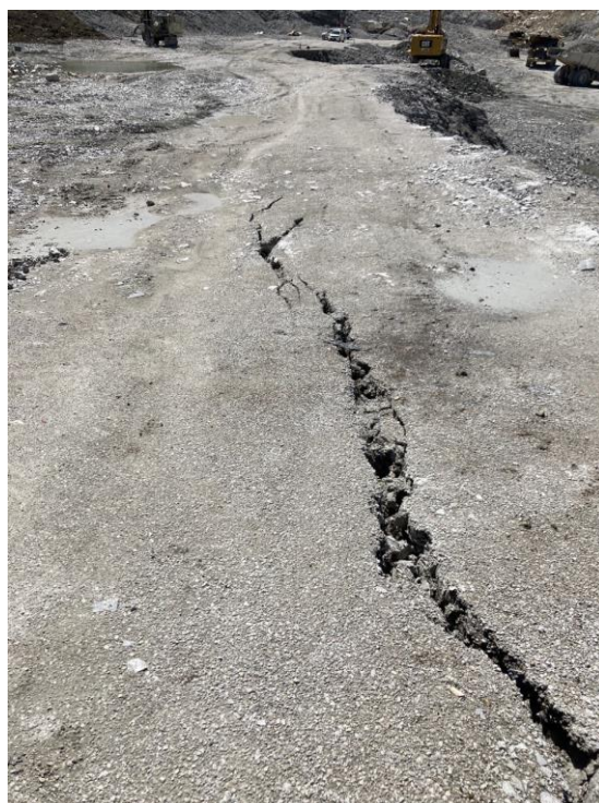
Fig.4.10 – Detail of tension cracks, July 2021.
