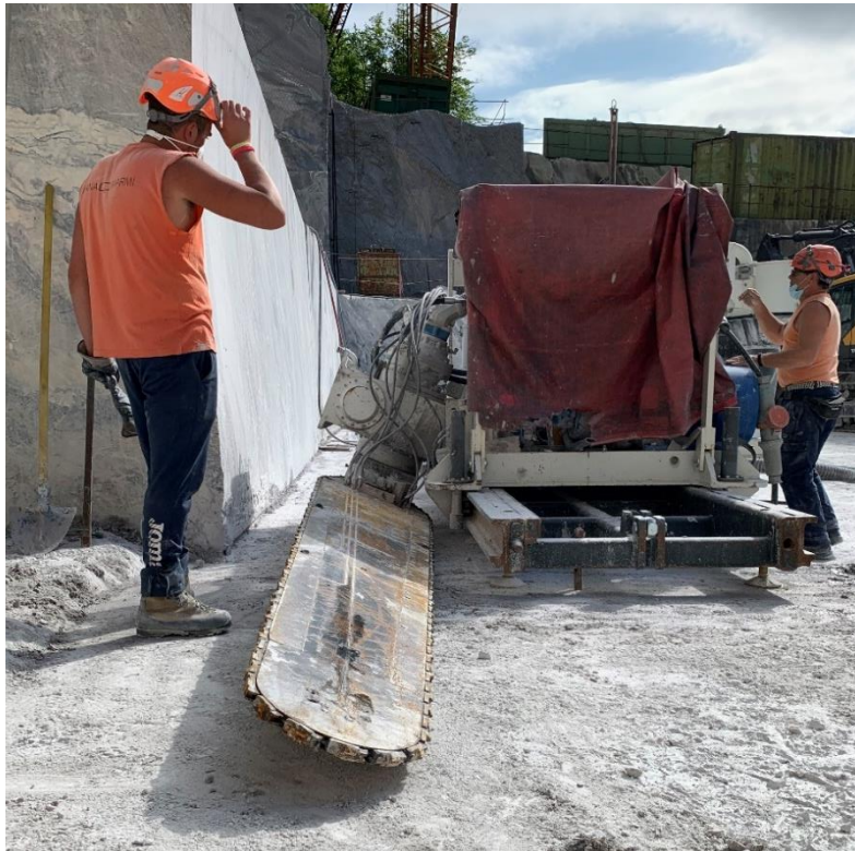
Figure 2.3 - Preparatory work of the chain saw cutting machine
