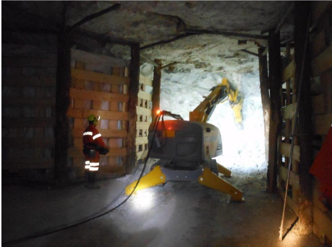
*Figura C3.6 -Robot martellatore “Brokk” all’opera<sup>36</sup>*
