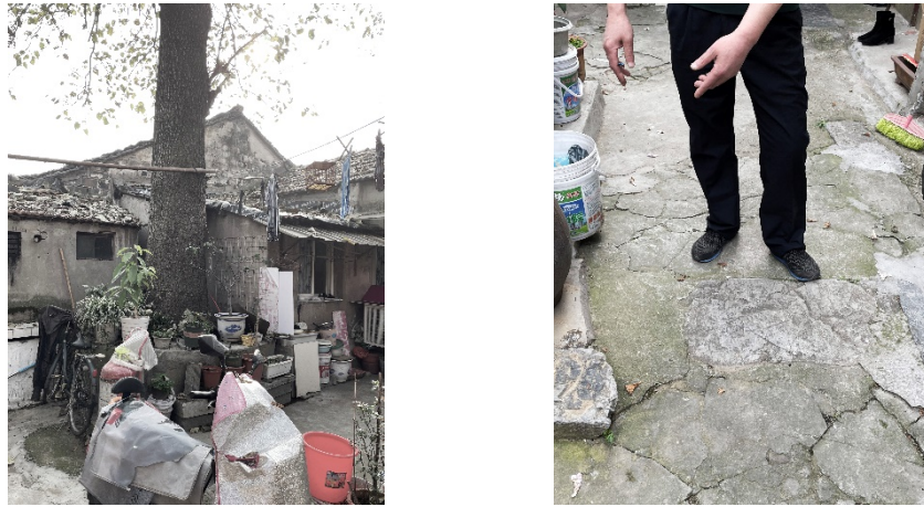
Figure 5-7 Walls and floors damaged by trees
