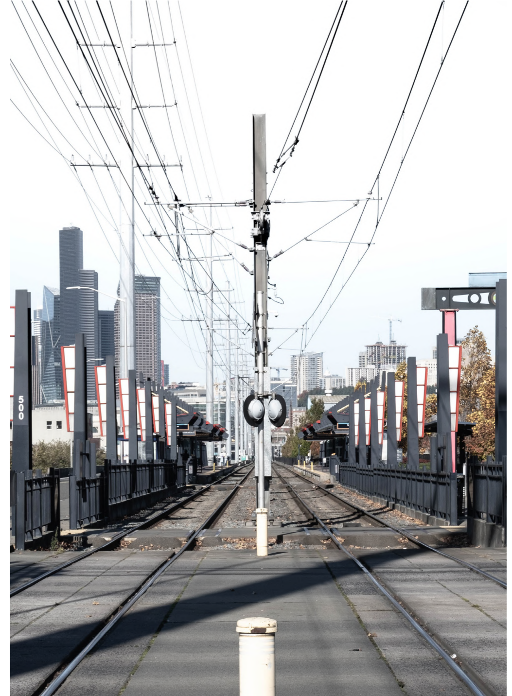
View of the SoDo Light Rail station from S Lander St looking north Daphne Fabbri ©2020
