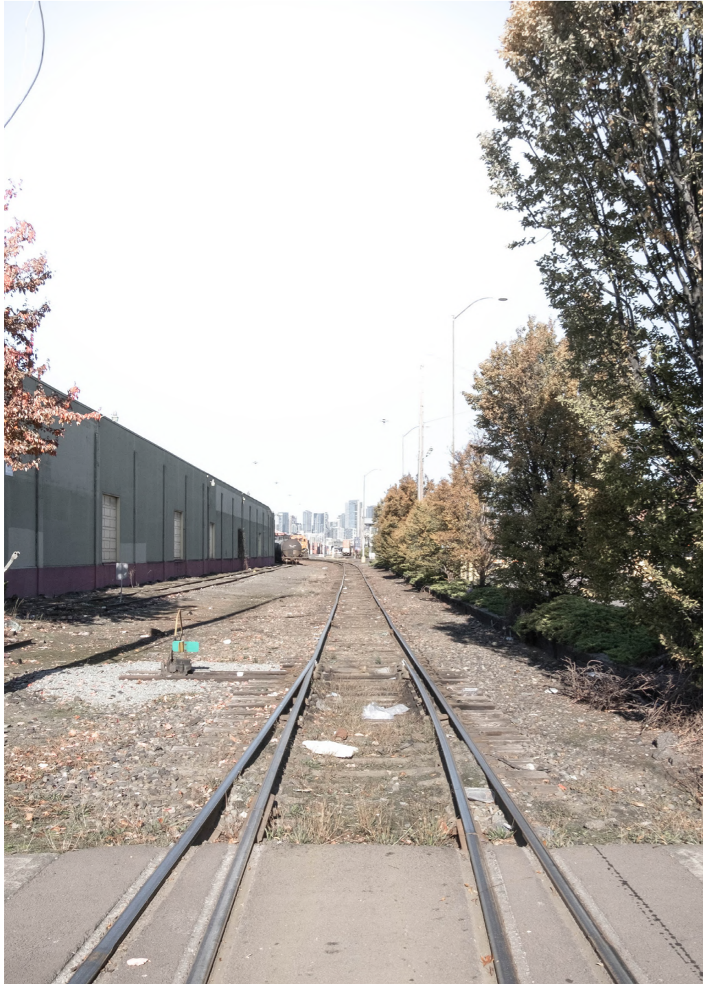
View of BSNF tracks from S Hanford St looking north Daphne Fabbri ©2020
