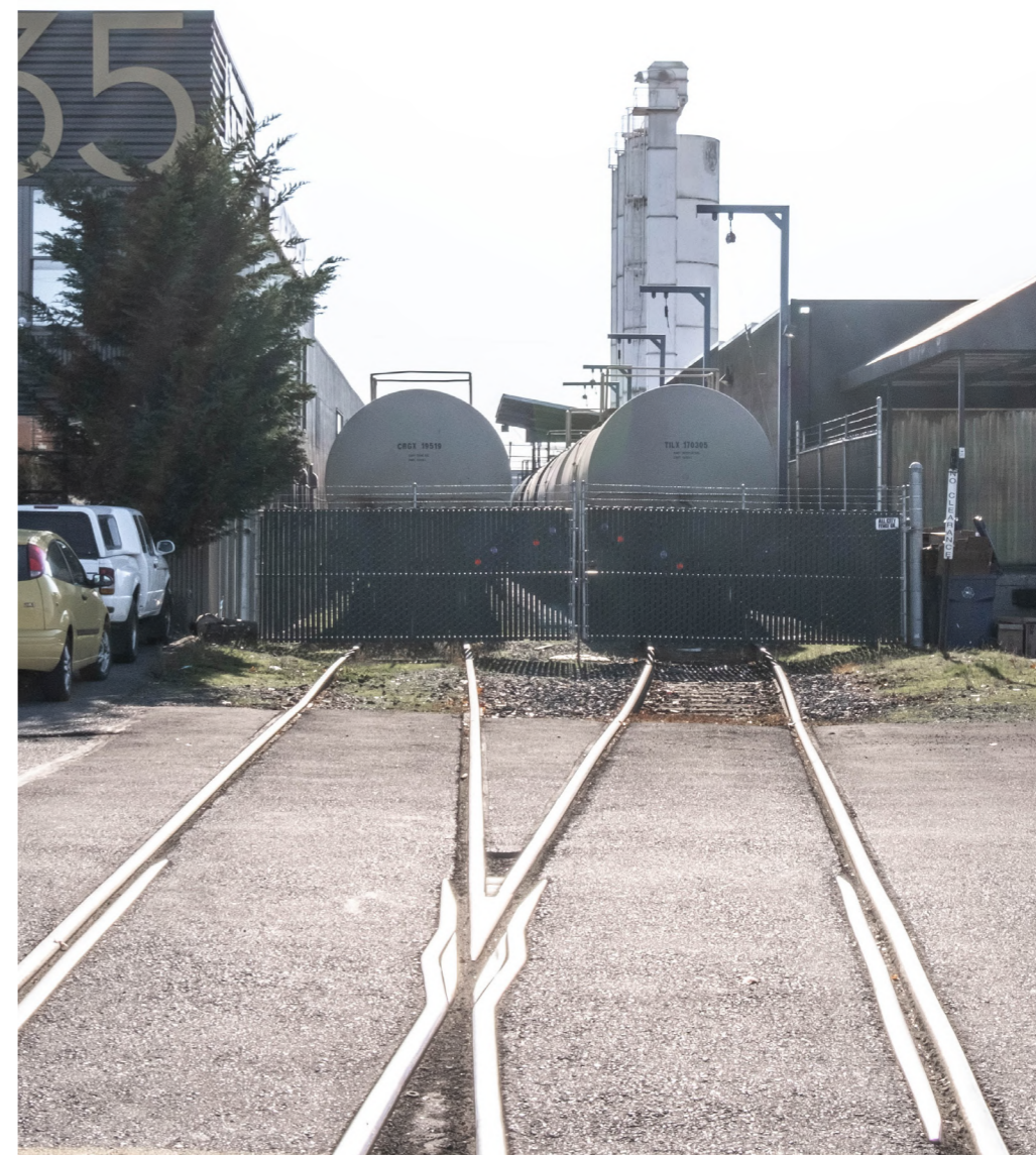
View of BSNF tracks from S Hanford St looking south Daphne Fabbri ©2020
