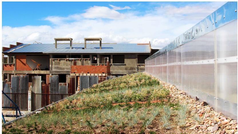
Figure 10. Final result of the extensive green cover
