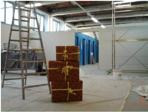
fig 4.10 bathroom before (fig by:www.casadelquartiere.it)
