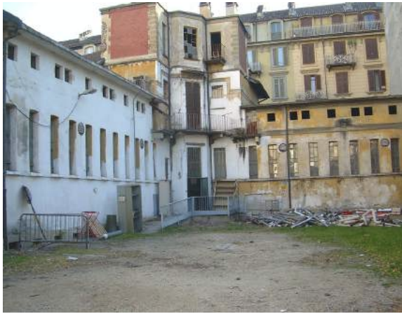
fig 4.16 courtyard before (fig by:www.casadelquartiere.it)
