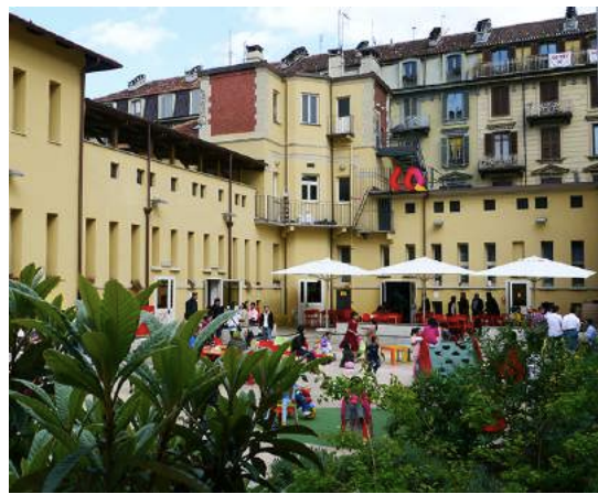
fig 4.17 courtyard after (fig by:www.casadelquartiere.it)
