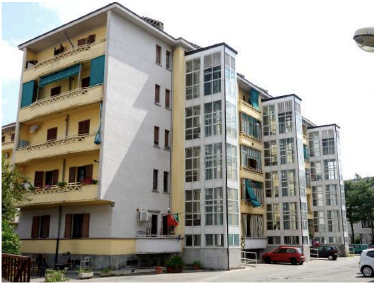
fig 5.26 elevator with consistent elevation (photo by author)
