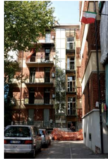
fig 5.27 translucent elevator (photo by author)
