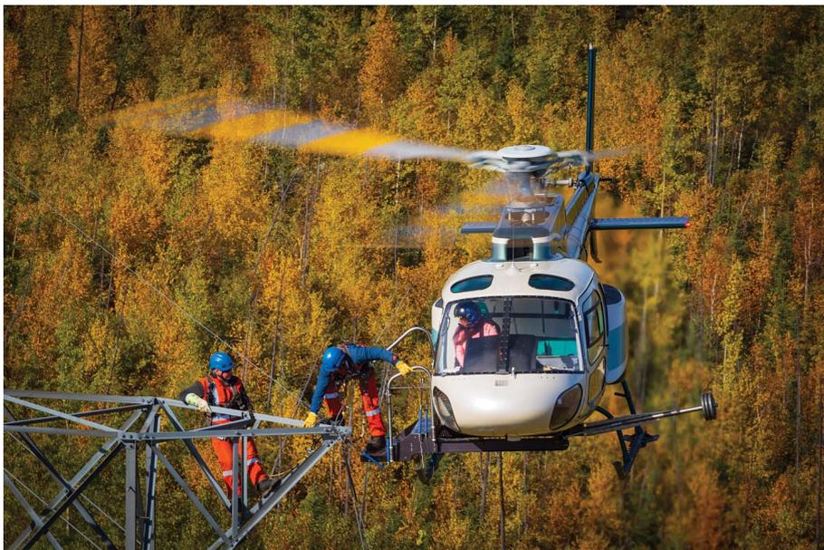
*Fig 1.2.3: Overhead Power Line maintenance operation*
