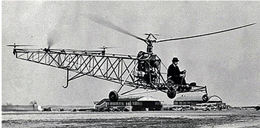
*Fig 1.1.2: VS-300 First Flight*
