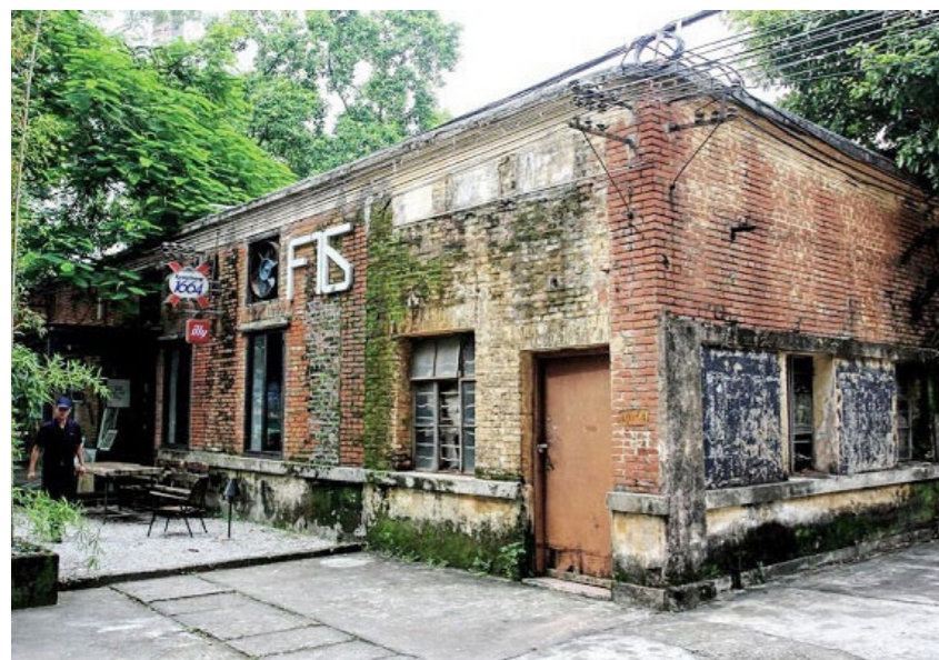
Figure 19 the transformed "red-brick" factory
