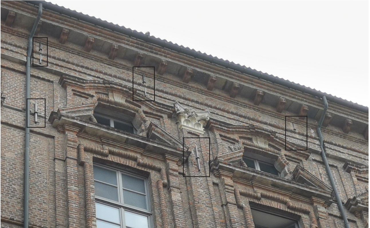
Fig.114 The metal bars exposed on the facade of Collegio dei Nobili
