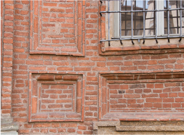
Fig.48 The framing of curved bricks on the facade of Palazzo Carignano
