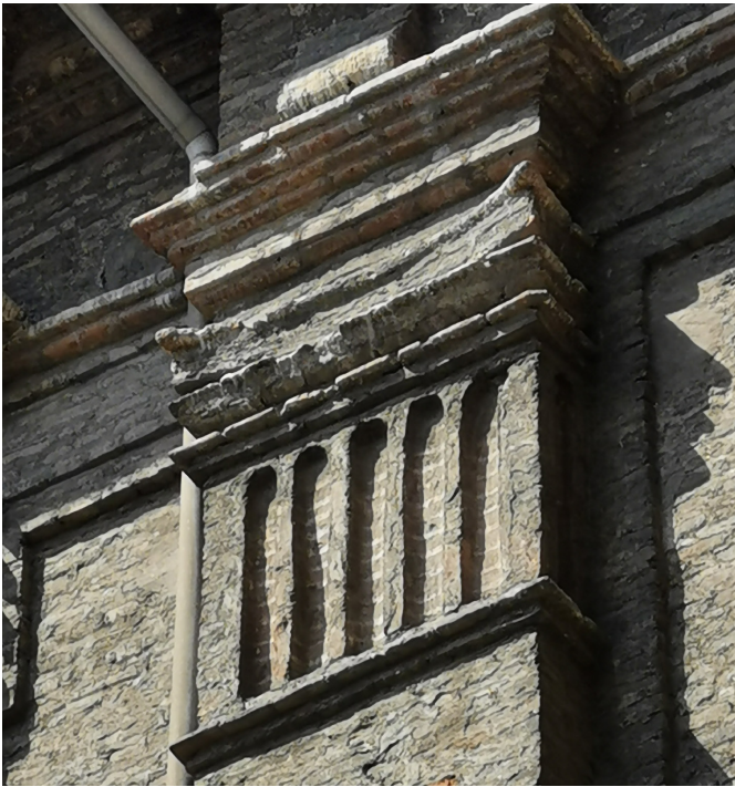
Fig.89 The upper structure on the pilaster of the Quartieri Militari, with the composite capital displaying triglyph-like vertical channels.
