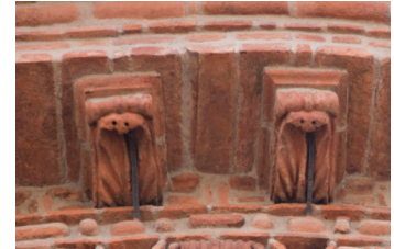
① modillions under the brick bedding course
