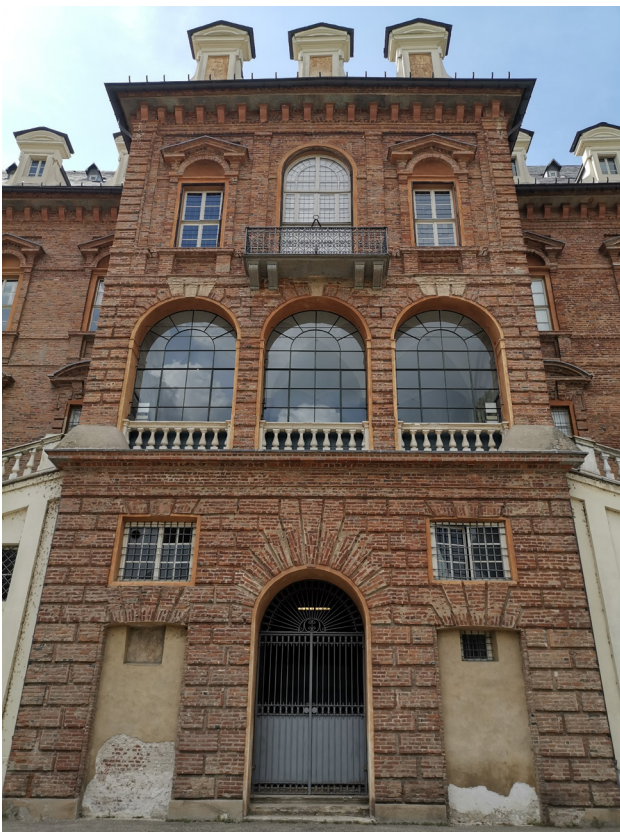
Fig.11 The protruding eastern facade of Castello del Valentino, with the portal, the three-arch loggia above it, followed by the windows and arched opening of the main building
