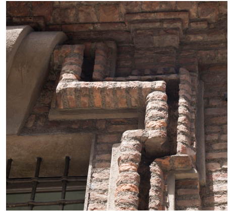
Fig.74 The mortar framing at both sides of the cylindrical brick frame
