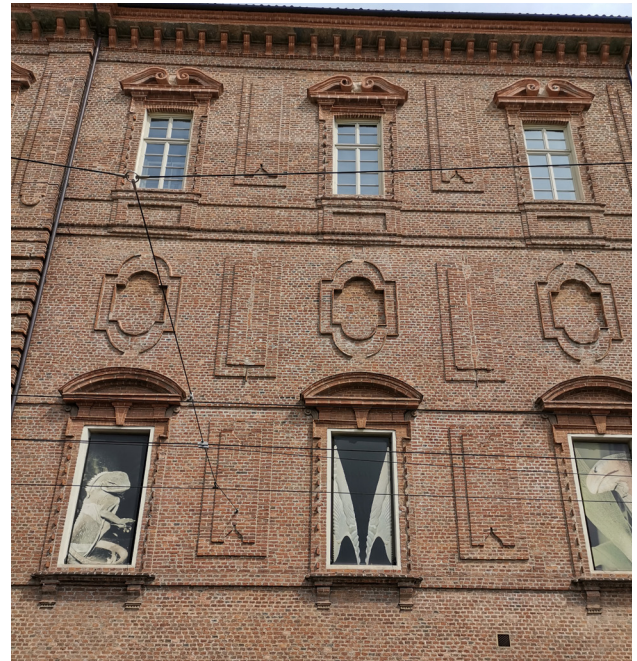
Fig.18 The string courses and brick ornaments dividing the western facade of the Ospedale di S. Giovanni
