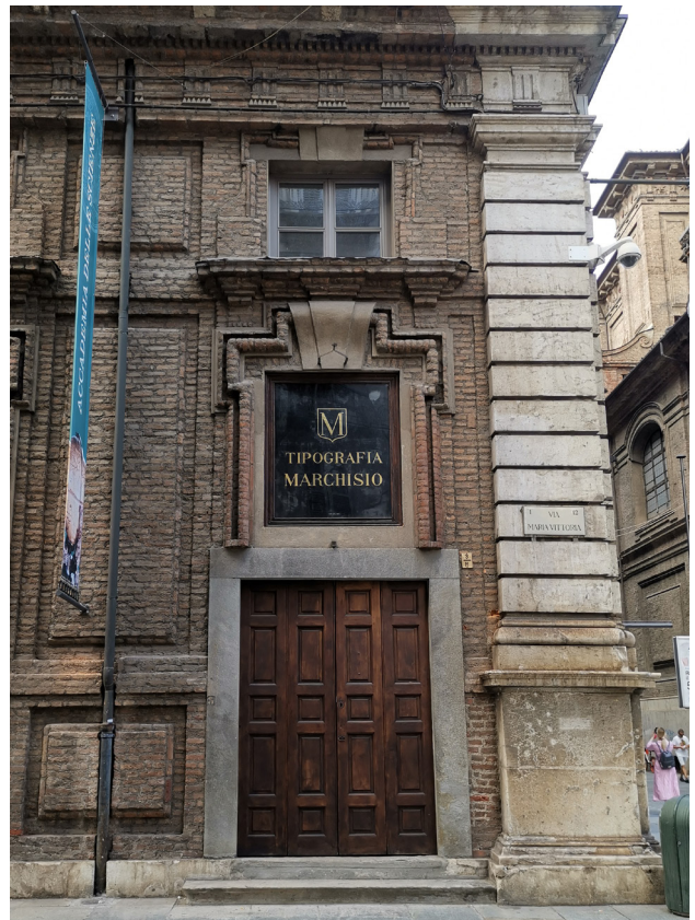
Fig.29 The door integrated with original window structure on the eastern facade of the Collegio dei Nobili
