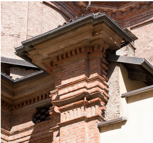
Fig.36 The pilaster, capital and entablature on the corner of the Chiesa di Santa Pelagia, making an elaborate assemblage
