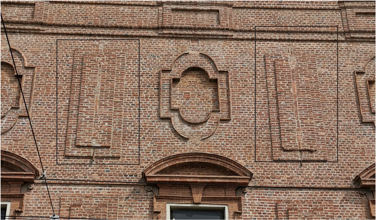
Fig.111 The metal bars located regularly on the western facade of the Ospedale di S.Giovanni, covered by segmental bricks with both ends exposed
