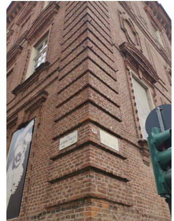
Fig.46 The rusticated brickwork at the corner of the Ospedale di S.Giovanni
