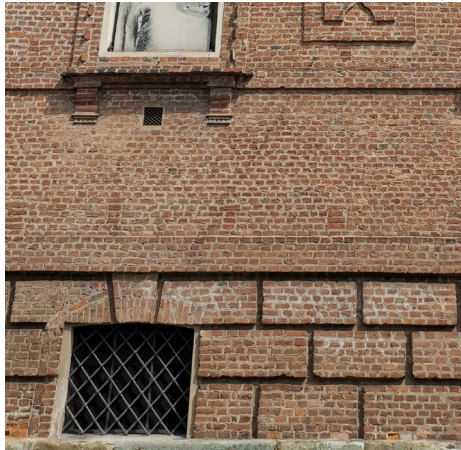
Fig.45 The rusticated brickwork at the base of the Ospedale di S.Giovanni
