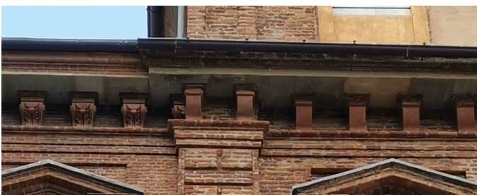
Fig.101 The cornice on the facade of the Castello del Valentino (the left part being the 19th-century terracotta corbels)
