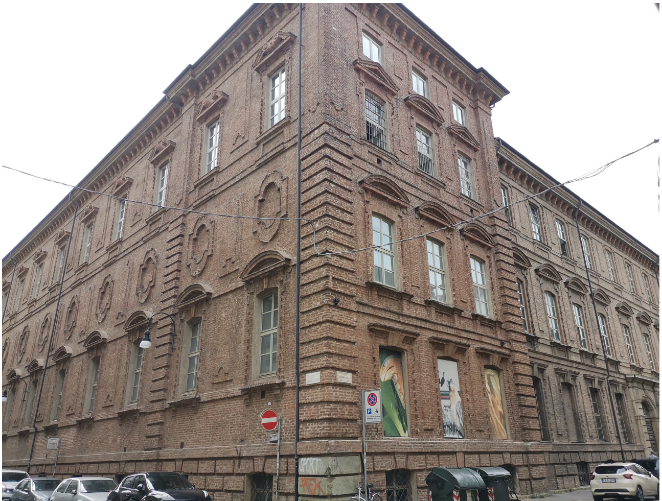
Fig.16 The north-eastern corner of the Ospedale di S.Giovanni, displaying the pavilion at the end of the eastern wing, also showing the different number of floors between the northern wing and the eastern wing
