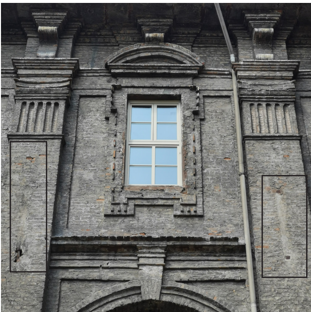
Fig.112 The metal bars hidden in the pilasters of the Quartieri Militari, with some exposed due to the falling off of pilaster
