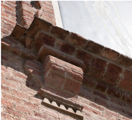
Fig.62 The triangular ornamental "guttae" at the window corbel on the western facade of the Ospedale di S.Giovanni
