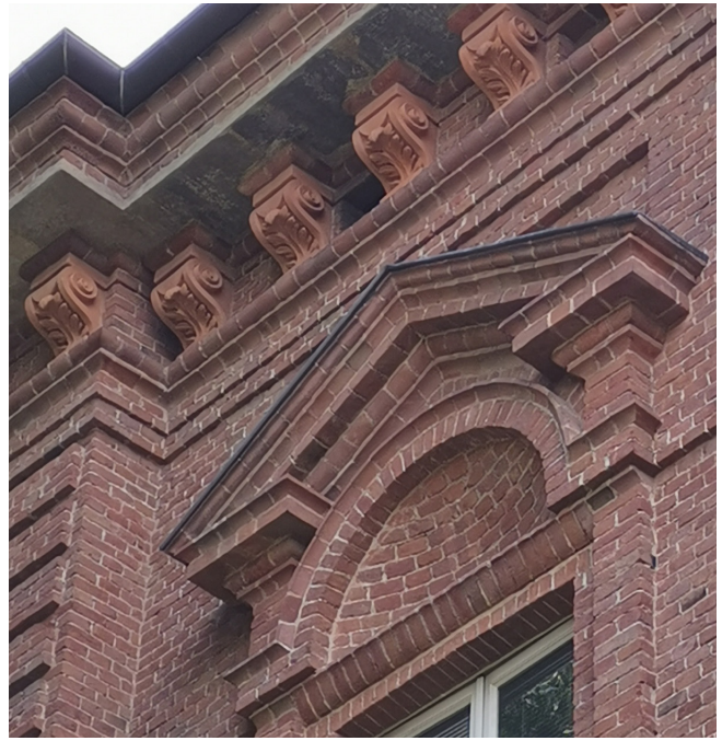
Fig.3 A part of the facade of Castello del Valentino, displaying the window pediment and cornice with special bricks used in the construction of the 19th-century facade
