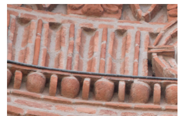
③ vertical channeling over "egg and dart" motif
