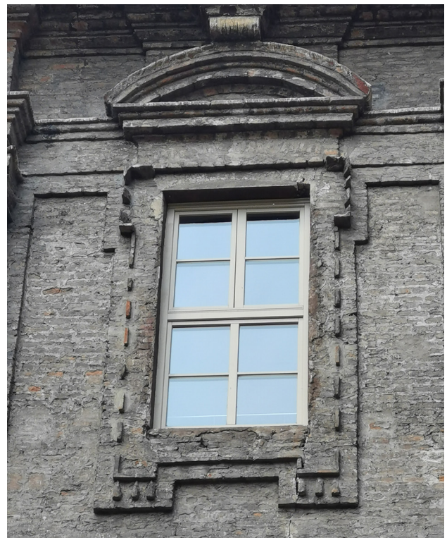
Fig.60 The window above the portico of the Quartieri Militari, with pointing out bricks and guttae
