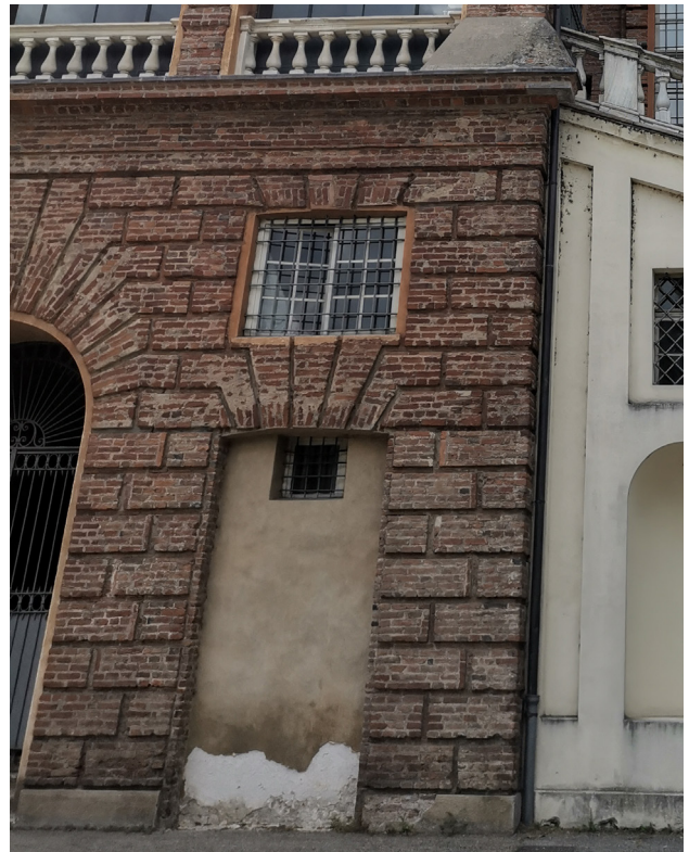
Fig.42 The "rusticated" brickwork on the eastern facade of the main building, emphasizing the portals and the corners
