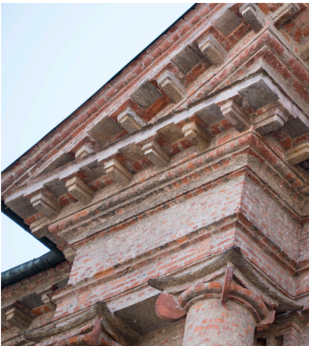
Fig.106 The cornice on the northern facade of the Chiesa di San Michele Arcangelo featuring stone modillions
