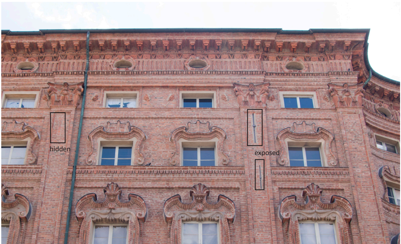
Fig.115 The metal bars on the western facade of the Palazzo Carignano
