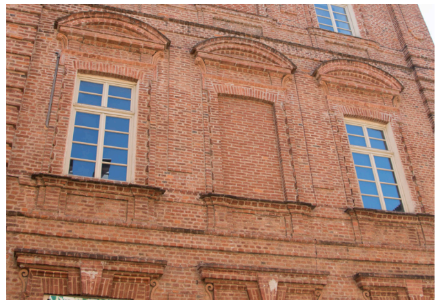
Fig.71 The large window bases integrated with string courses of the first-level windows on the northern facade of the Ospedale di S.Giovanni
