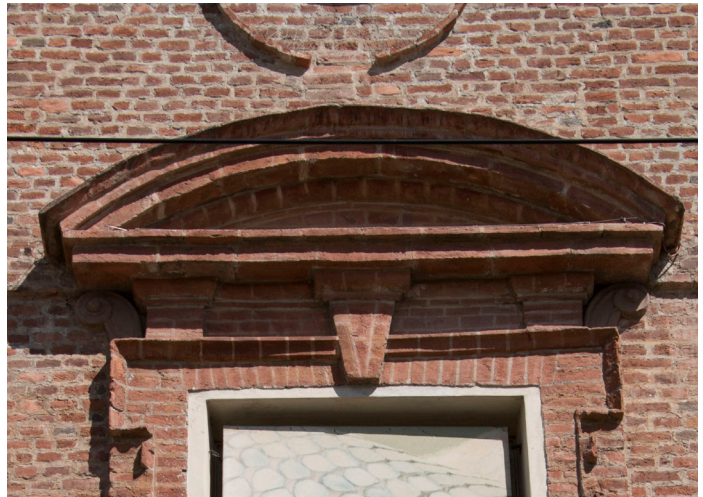
Fig.64 The flat arch on the ground-floor window of the western facade of the Ospedale di S.Giovanni
