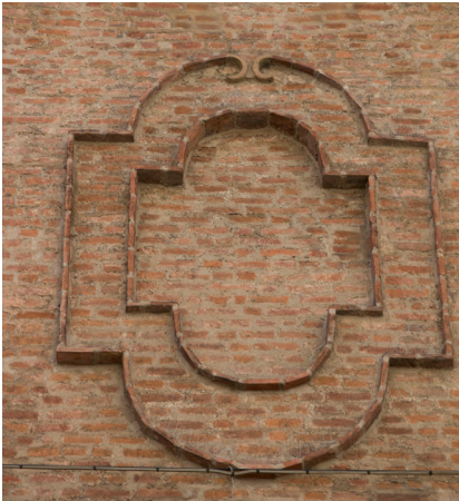
Fig.44 The ornamental projecting bricks on the facade of Ospedale di S.Giovanni
