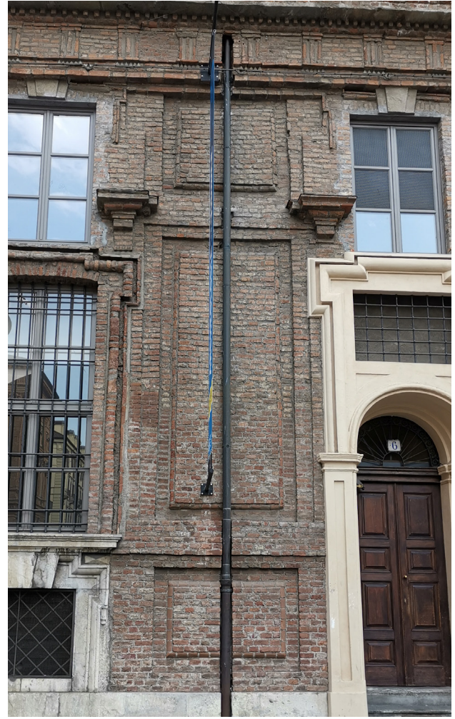
Fig.50 The framing of curved bricks on the facade of Collegio dei Nobili
