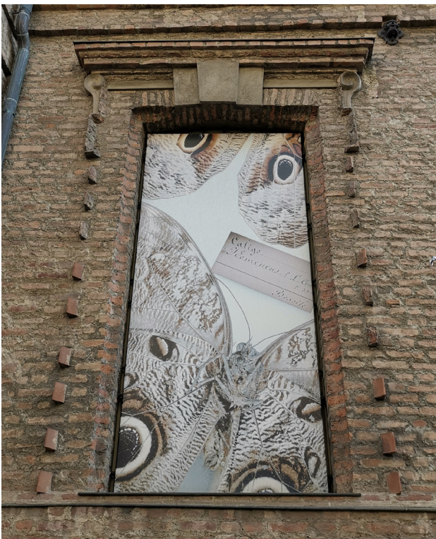
Fig.59 The 17th-century window on the northern facade of the Ospedale di S.Giovanni, with pointing out bricks surrounding the frame
