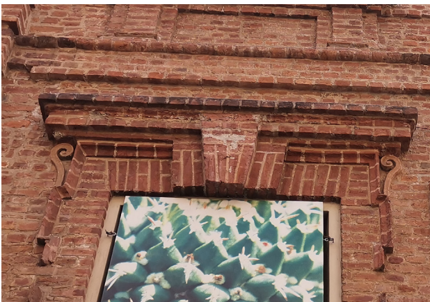
Fig.70 The "keystone" brickwork of the northern facade window of the Ospedale di S.Giovanni
