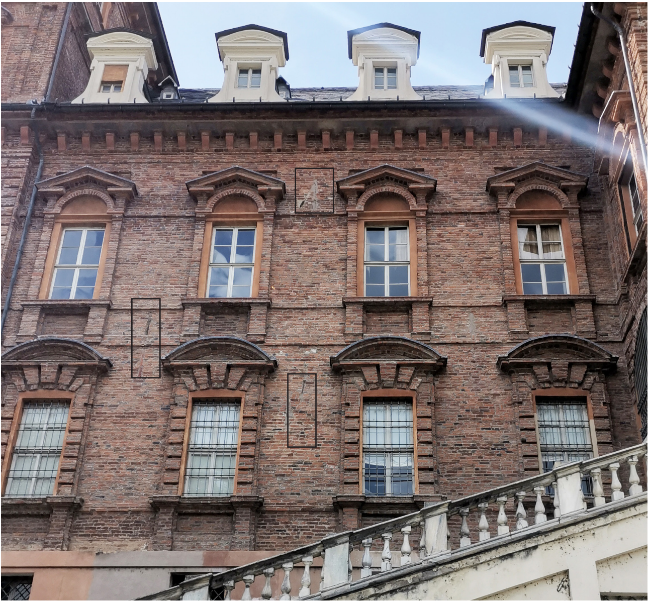
Fig.110 The visible metal anchor rods on the 17th-century facade of the Castello del Valentino
