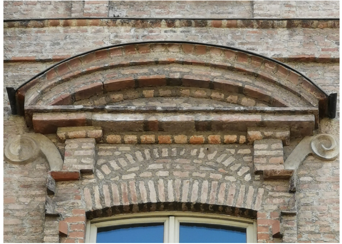
Fig.63 The segmental arch and relieving arch on the first-floor window on the northern facade of the Ospedale di S.Giovanni
