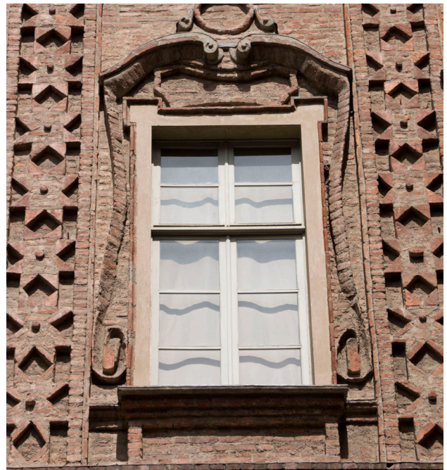
Fig.83 The baroque window on the courtyard facade of the Palazzo Carignano, with the curtain-like frame on its sides, made of moulded and sculpted bricks
