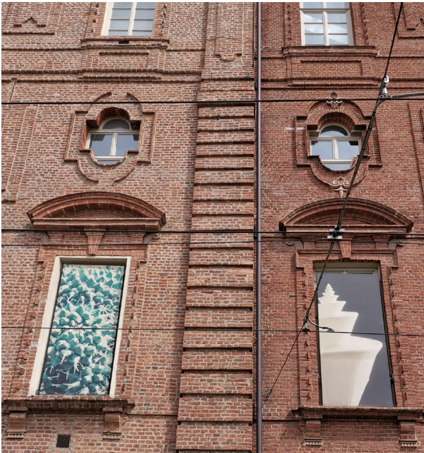
Fig.17 The two parts of the western facade with the same brickwork but brick of different size
