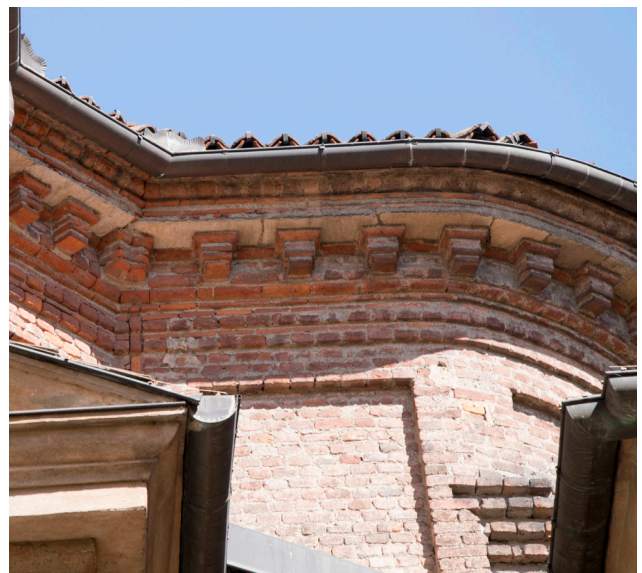
Fig.107 The cornice on the western facade of the Chiesa di Santa Pelagia featuring rectangular brick modillions
