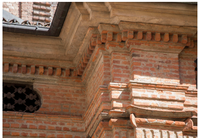
Fig.108 The brick-only lower cornice on the western facade of the Chiesa di Santa Pelagia featuring blocks of brick as dentils
