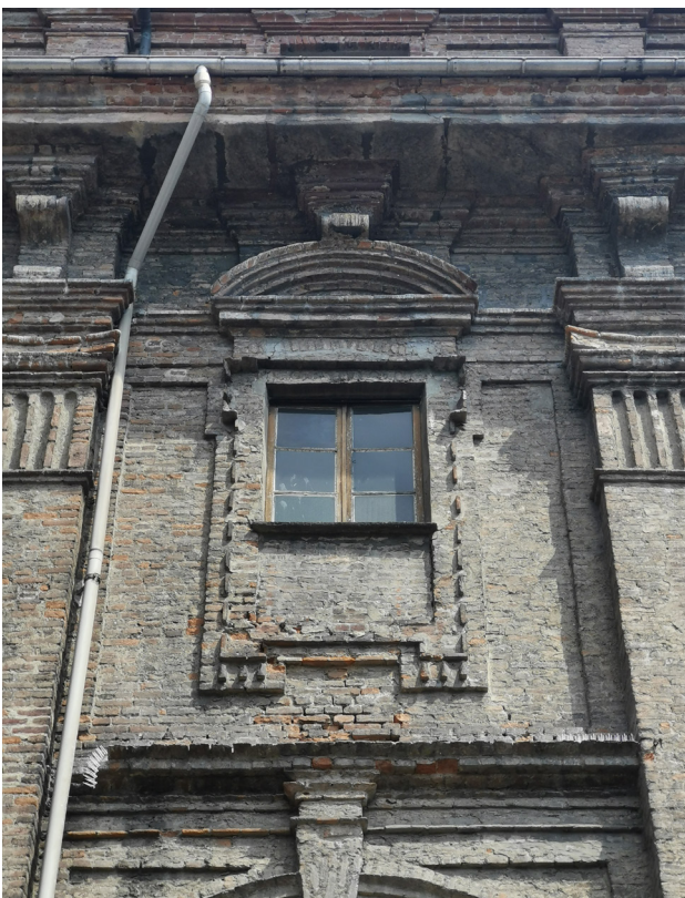
Fig.33 The window partly filled with bricks above the portico of the Quartieri Militari
