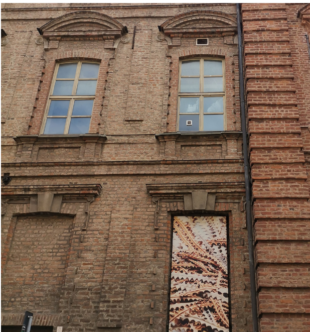
Fig.19 The windows on the northern facade of the Ospedale di S. Giovanni which have been repeatedly modified
