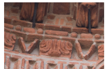
② moulded/cast brick
