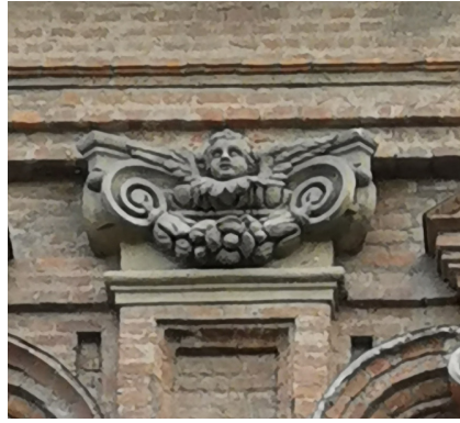
Fig.86 The stone capital on the first-level order of the Collegio dei Nobili
