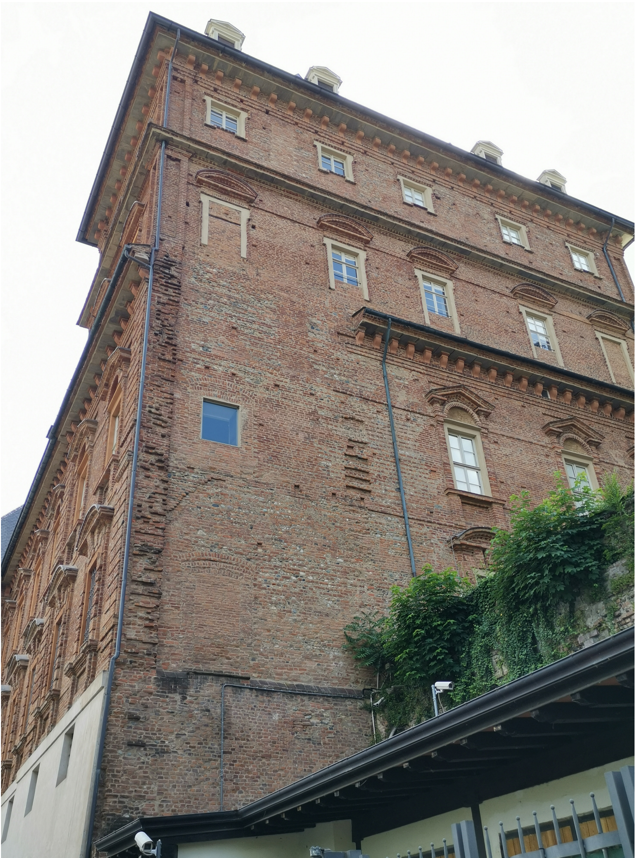
Fig.14 The northern facade of the Castello del Valentino, displaying the wall that was supposed to connect the incomplete northern wing.
