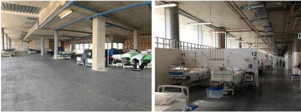
Picture 2. Hospital del Mar before and after the reconversion of the ground floor.
