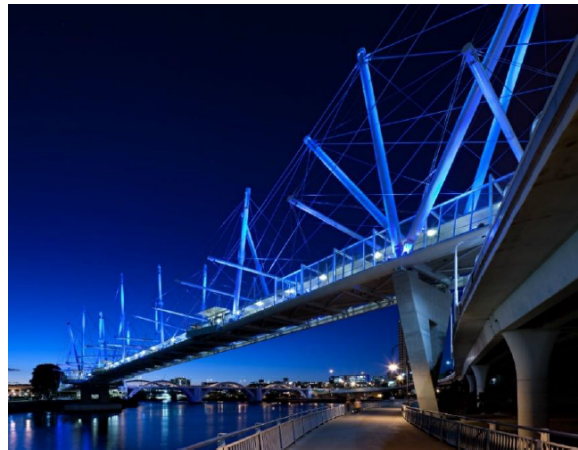
Figure 3.4: Kurilpa Bridge, Brisbane, Australia. Source [20]
