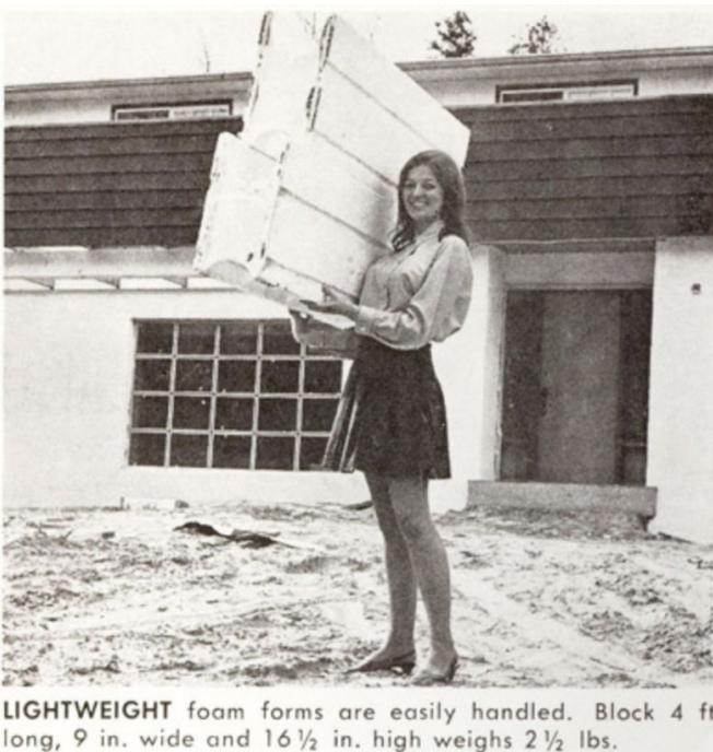
LIGHTWEIGHT foam forms are easily handled. Block 4 ft long, 9 in. wide and 16 1/2 in. high weighs 2 1/2 lbs.
