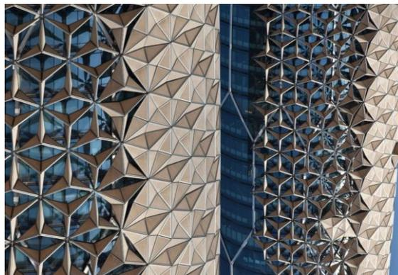
Fig. 41: Al Bahr towers shading system
