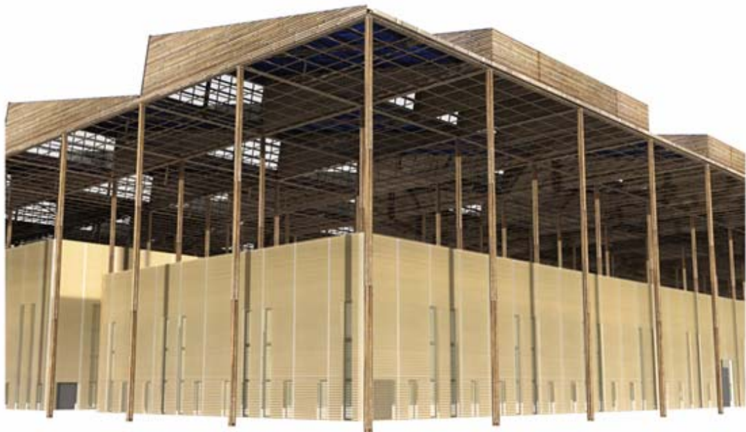
Bamboo bearing structure of the covering
