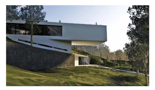
Due to the quite large prolongation, the third level of the museum is constituted of a reticular structure, inserted into two huge reinforced concrete slabs. It will be made of a metallic section, especially of HEA beams, directed transversally to the projection, and a bigger beam directed diagonally to be sustained by the supporting wall below, at the second level.
