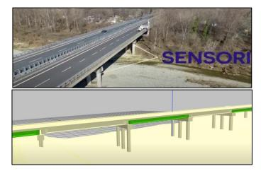
Figure 18. Location of the sensors previously position on the Stura Bridge and the model created. Source: ANAS S.p.A. and SYSDEV – Monitoraggio struttrale di ponti e viadotti.
