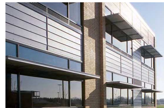
[53] AHMAD ELTAWEL, YUEHONG SU, Evaluation of Suitability of a Parametrically Controlled Louvers for Various Orientations throughout a Year Comparing to an Existing Case , Buildings 2017, Volume 7(4).
