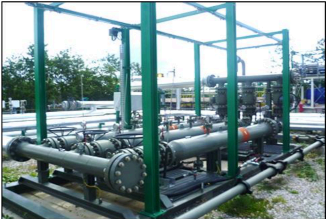
Figure 3.14 Triple Sand Catcher
