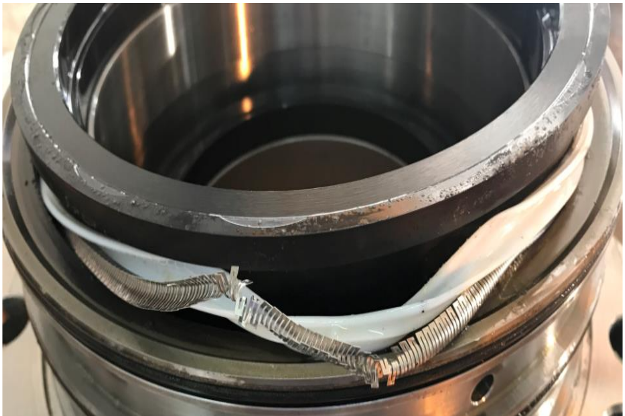
Figure 3.9 Stationary ring gasket completely damaged
