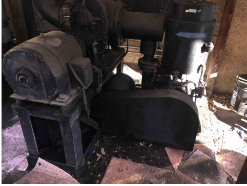
(a) Mechanical roughing pumps
