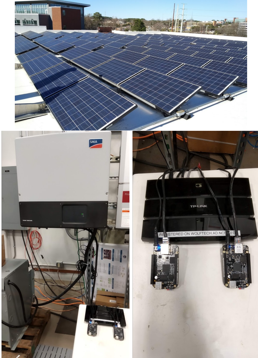
Figure 5.14. Solar panels (a), Inverter SMA STP-20000TL-US-10 (b), Router and BBBs connections (c)
