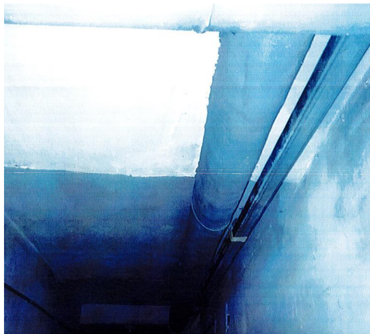
Figure 24: Insulating pipes containing friable asbestos [43]
