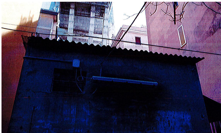
Figure 23: Example of roof in asbestos cement [44]
