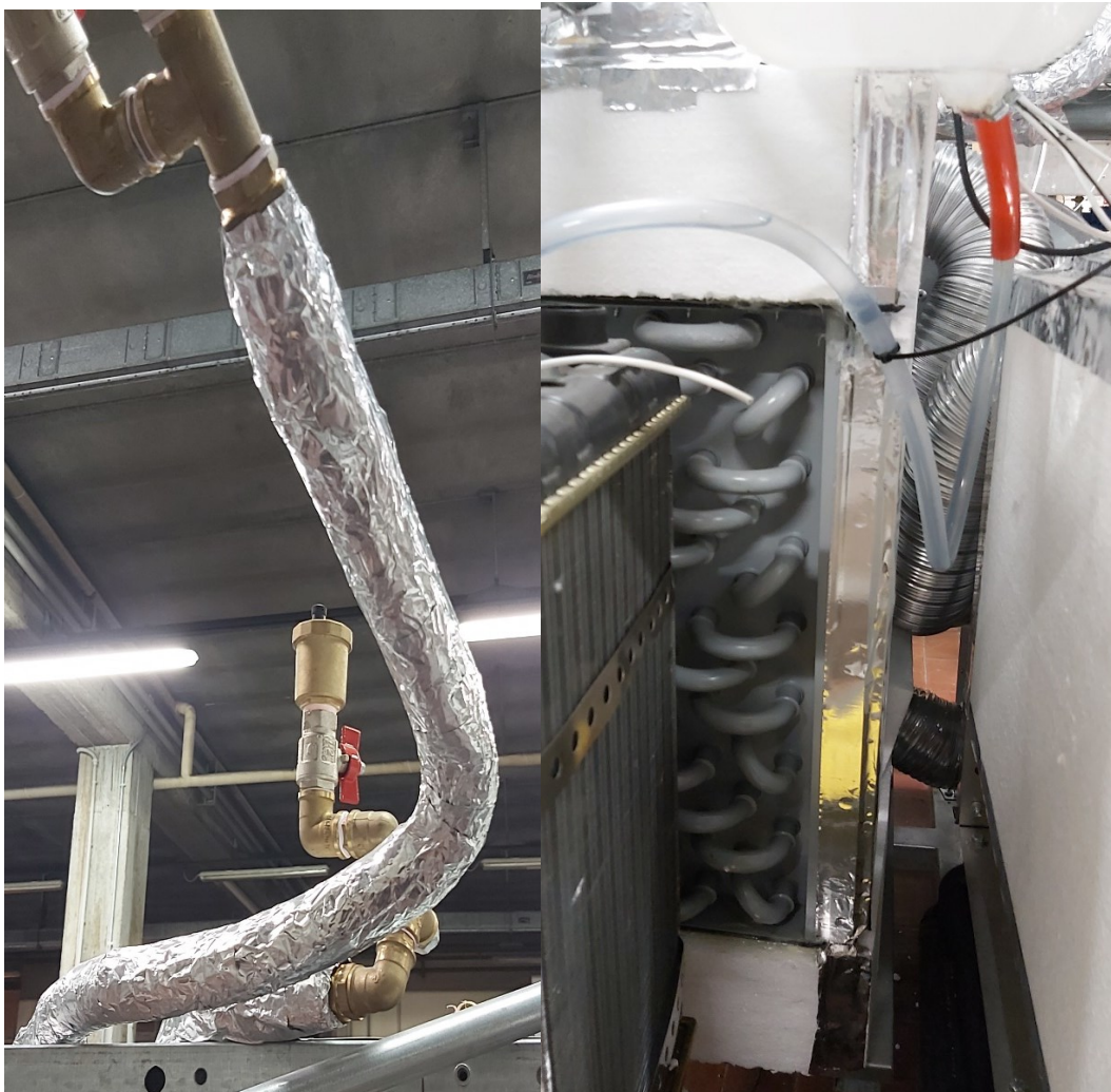
Figure 32. Insulation of the condenser
