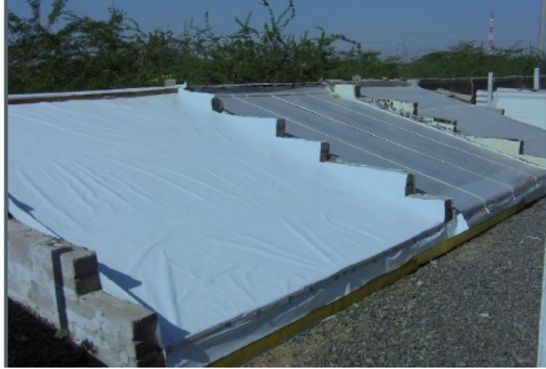
Figure 7. Pilot dew condenser at Kothara (Northwest India) [21]
