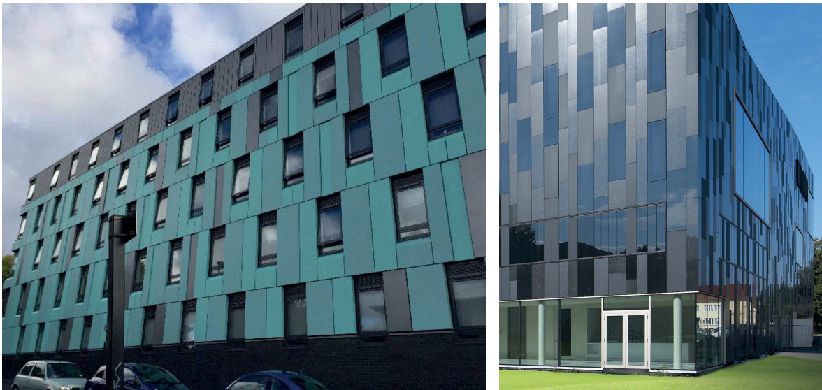
Fig. 1.9 Lightweight panels cladding system (Url 9,10)
