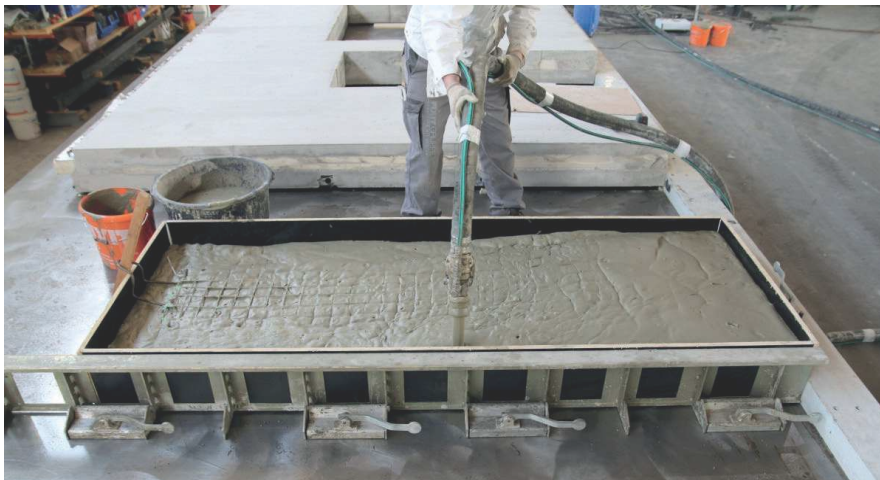
Fig. 1.22 Precast concrete is vibrated and levelled (Url 12)
