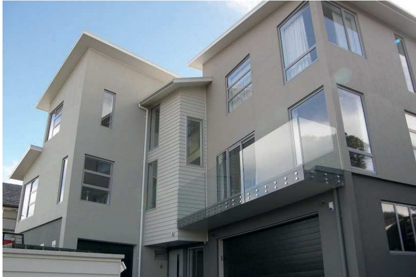
Fig. 1.7 Monolithic cladding cladding system (Url 7)
