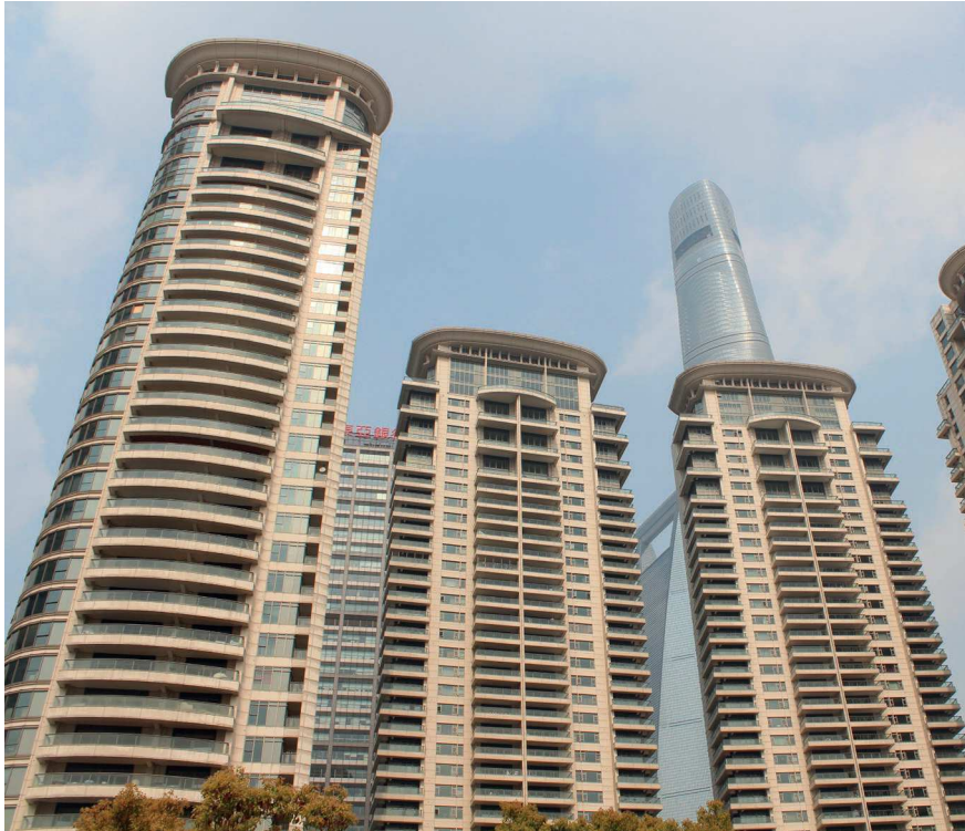
Fig. 1.10 Heavy panels cladding system (Shanghai,2019)
