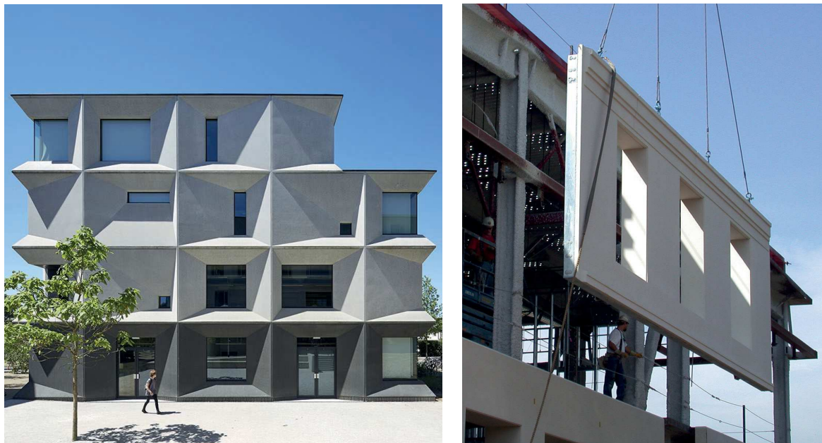
Fig. 1.25 Examples of window wall units (Url 16 -17)
