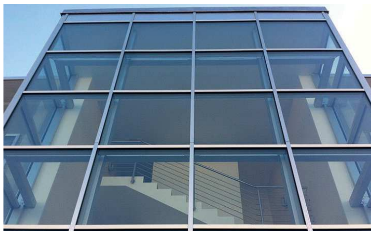
Fig. 1.2 Curtain wall cladding system: stick curtain (Url 4)
