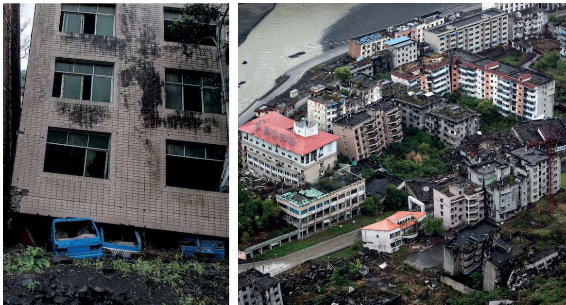
Fig. 4.1 The tragic consequences of 7.9 magnitude earthquake in Sichuan Province, 2008 (Url 22-23)
