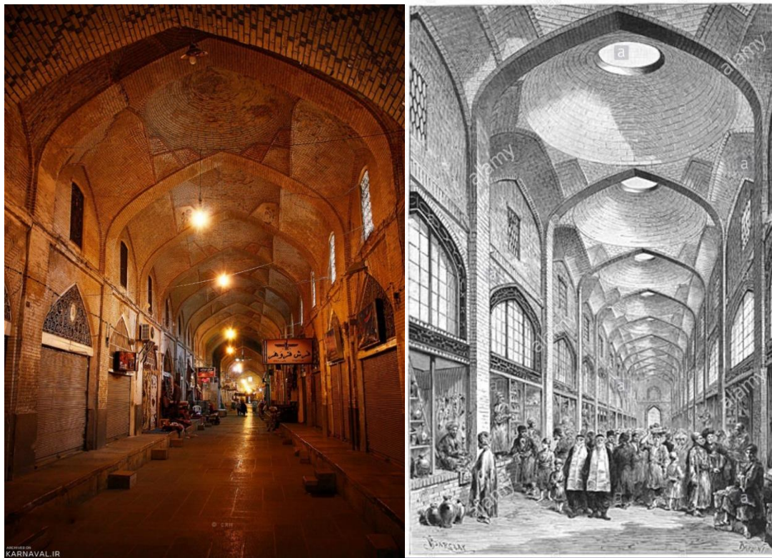
Figure 60. Materials of Vakil Bazaar include stone for foundation and brick for vaulted roof. In the right photo, the windows above the shops and holes in the vaulted roof are visible. (left photo by www.Shirazblog.com , 2019. Accessed November 24, 2019) Right photo Vakil Bāzār of Shiraz as seen by :Jane Dieulafoy in 1881. [ http://www.gutenberg.org/files/13901/13901-h/13901-h.htm Project Gutenberg]. <br />,2009 Accessed November 24, 2019)
