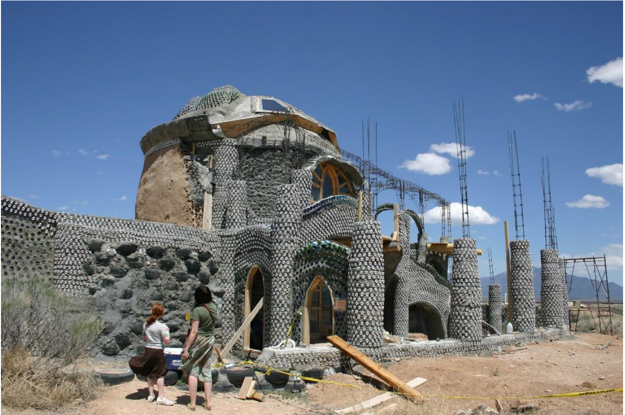
Figura 6 – Earthship Biotecture Project
