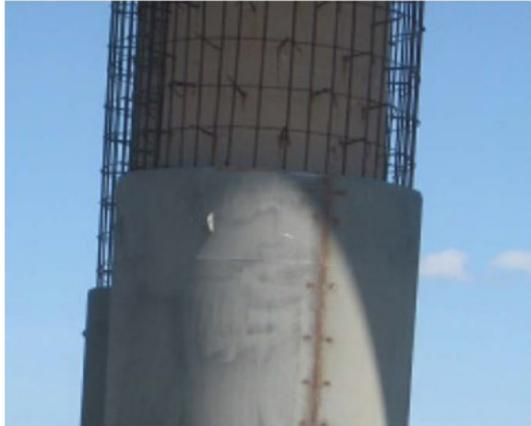
Figure 7.7: Concrete overlays along with an external reinforcement around the column [47]
