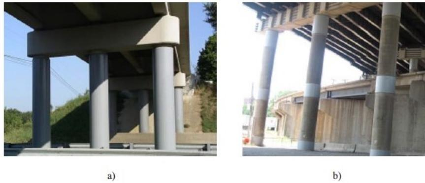
Figure 7.5: (a) Full column steel jacketing used in Tennessee, (b) partial height steel jacketing in Missouri focusing in plastic hinge regions of the columns [47]
