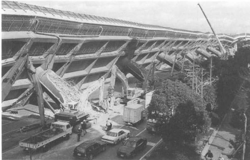
Figure 7.1: Flexural failure above the columns base of the Hanshin expressway during 1995 Kobe earthquake
