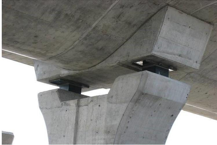
Figure 2.11: Detail of the application of neoprene bearings
