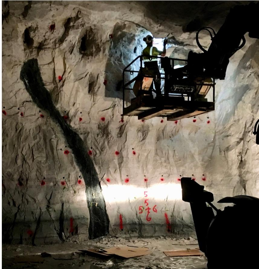
Figure III.6 Charging of the roof holes
