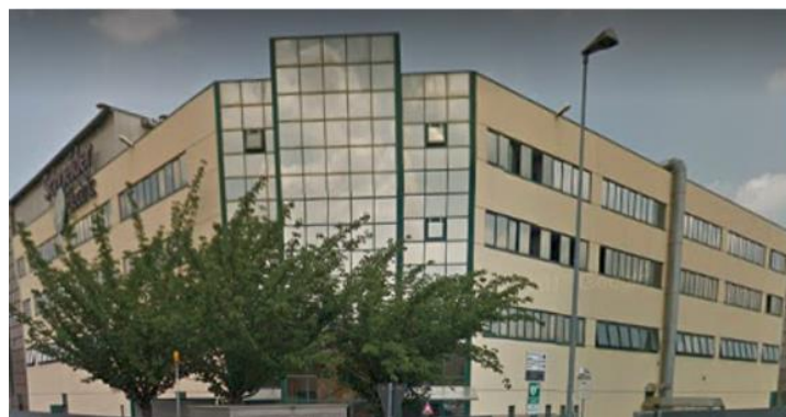
Figure 5 Schneider Electric distribution centre in Venaria 12
