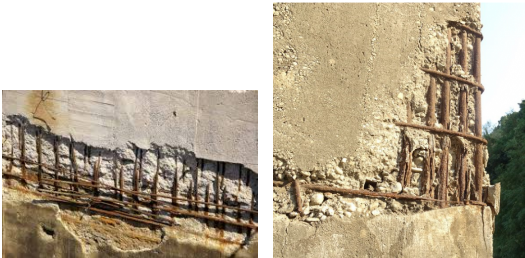
Figure 1.7: Corrosion in reinforced concrete structures
