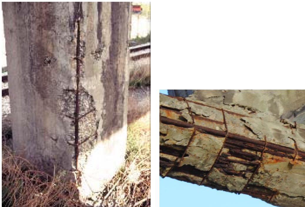
Figure 5.1: Cover detachment after corrosion of steel reinforcement
